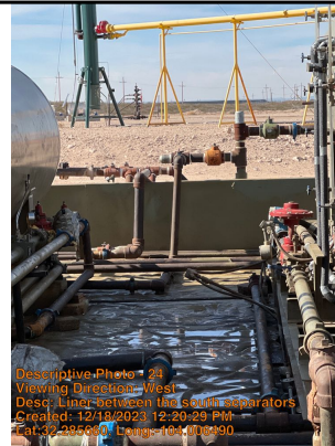
Liner between the south separators
