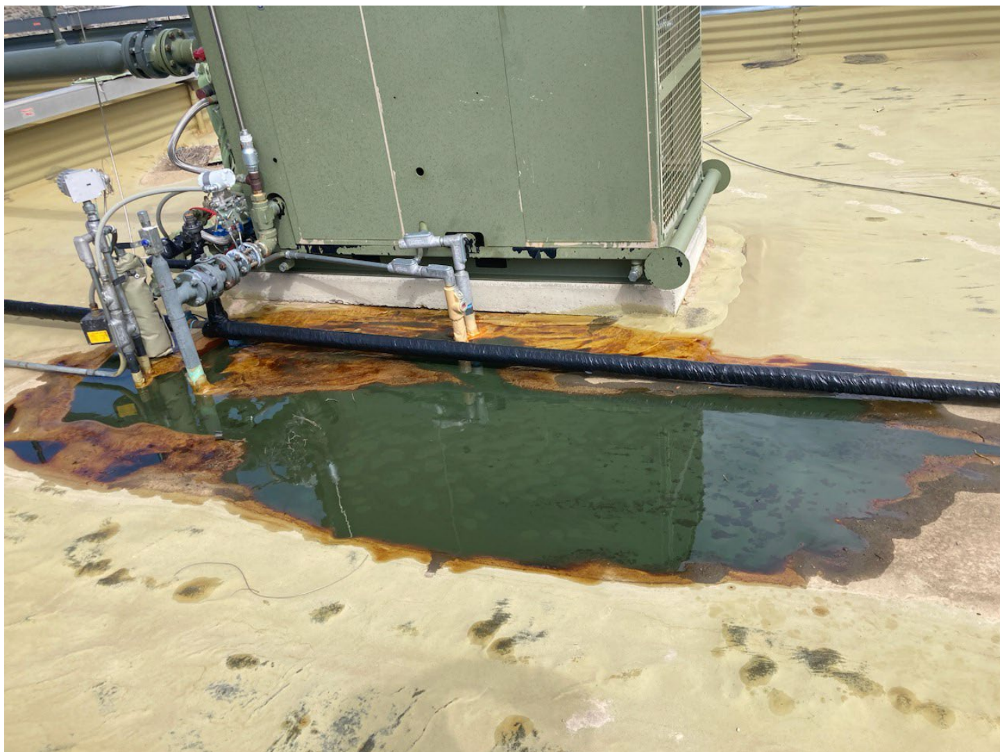
NE Lybrook Com 191 H oil tank leak. 3-31-24 where oil came up from under the liner. (29.6 bbl)
