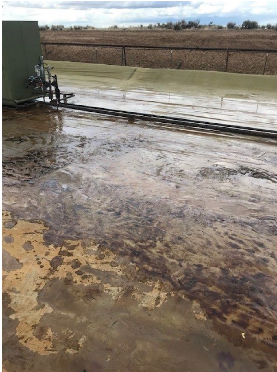
Produced water on liner prior to cleanup.
