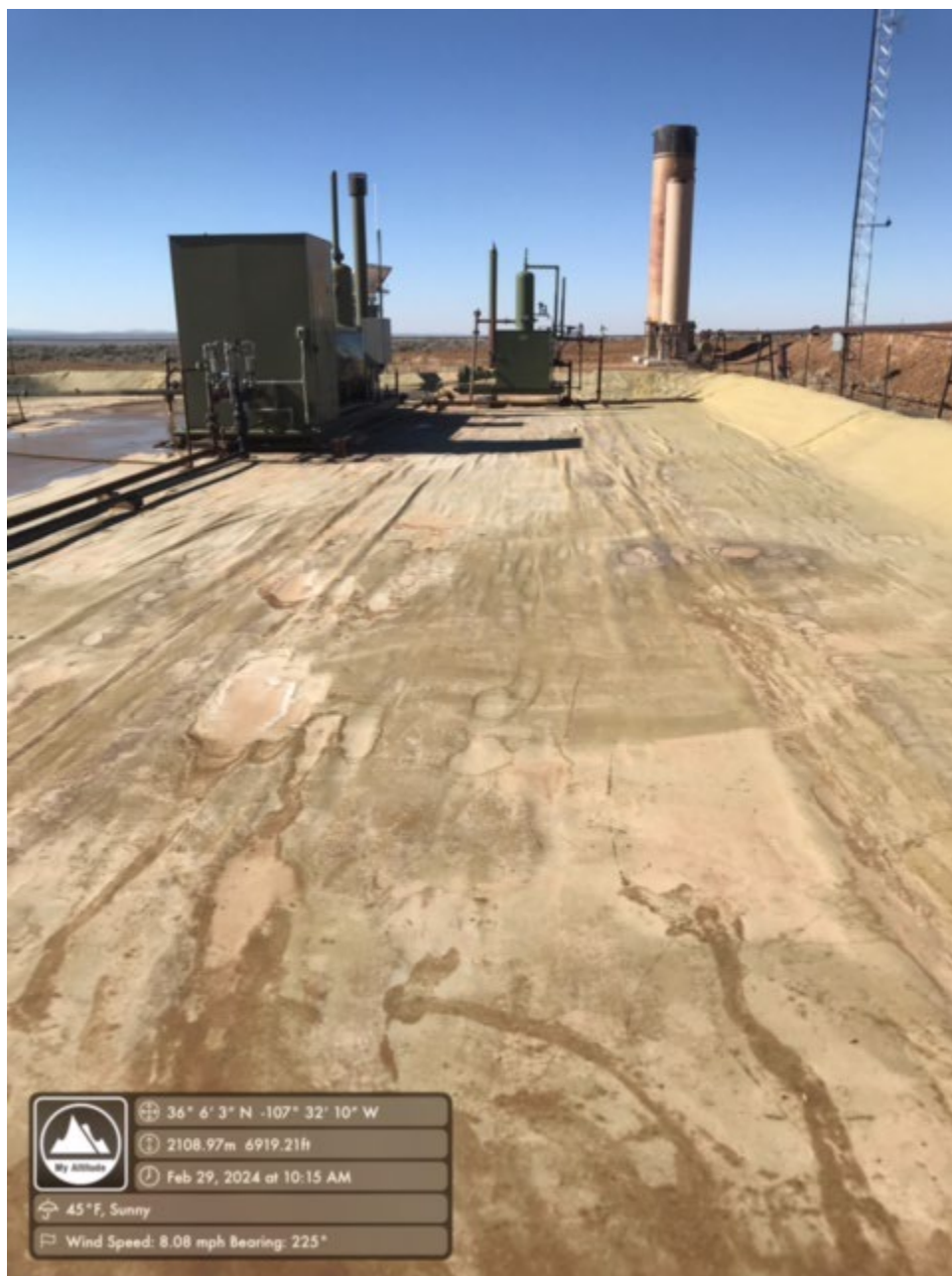
Liner inspection after replacing the Burner tube and liner cleaning.
