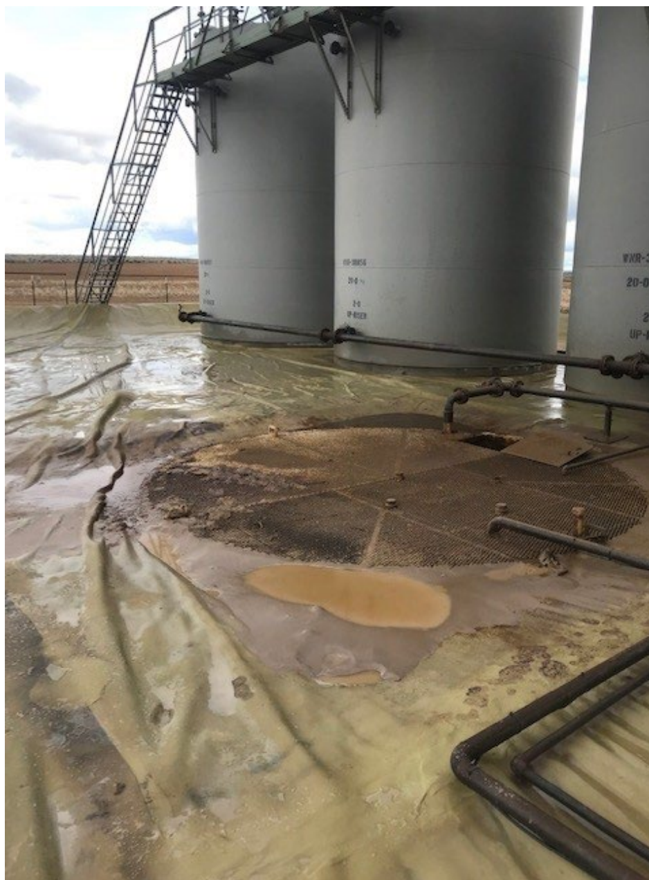
Produced water on liner prior to cleanup.
