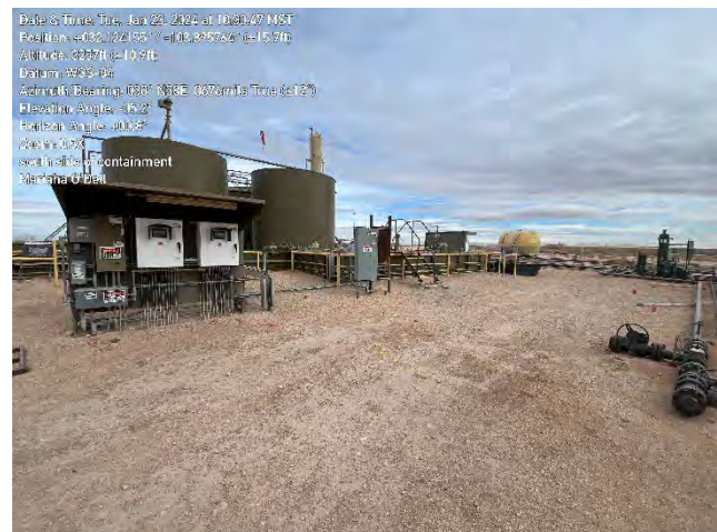
Photograph 4 Date: 1/23/2024 Description: Active equipment surrounding active, lined containment. View: Northeast
