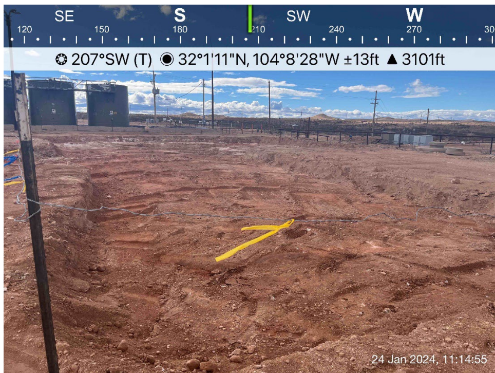
Excavated area viewing southwest, January 2, 2024
