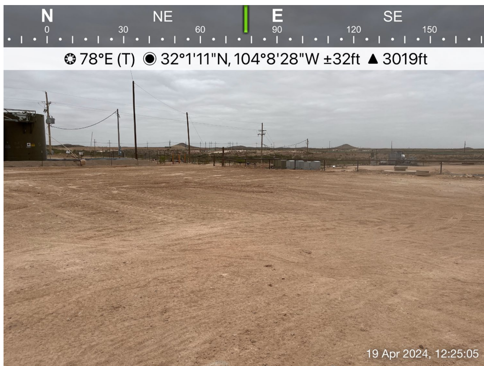
Backfilled excavation viewing east, April 15, 2024
