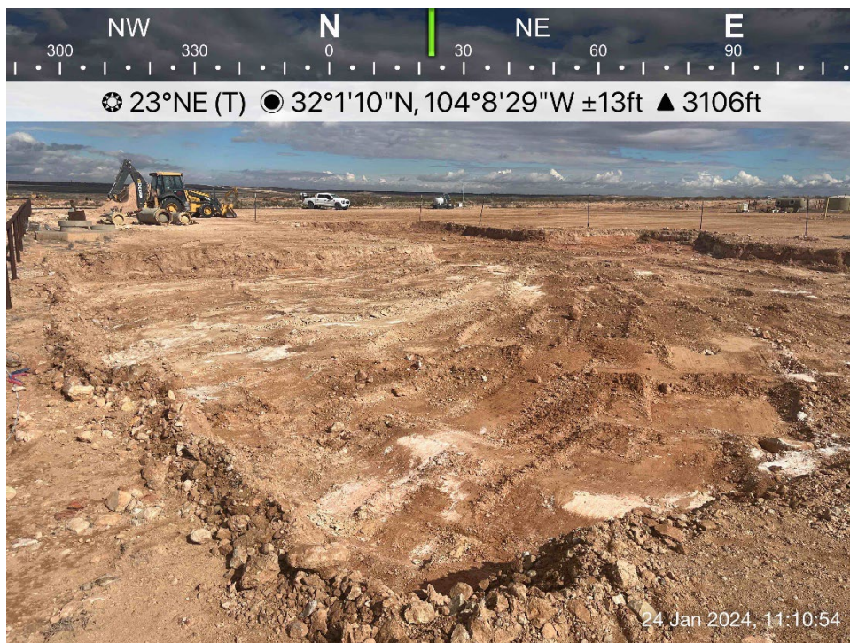
Excavated area viewing northeast, January 24, 2024
