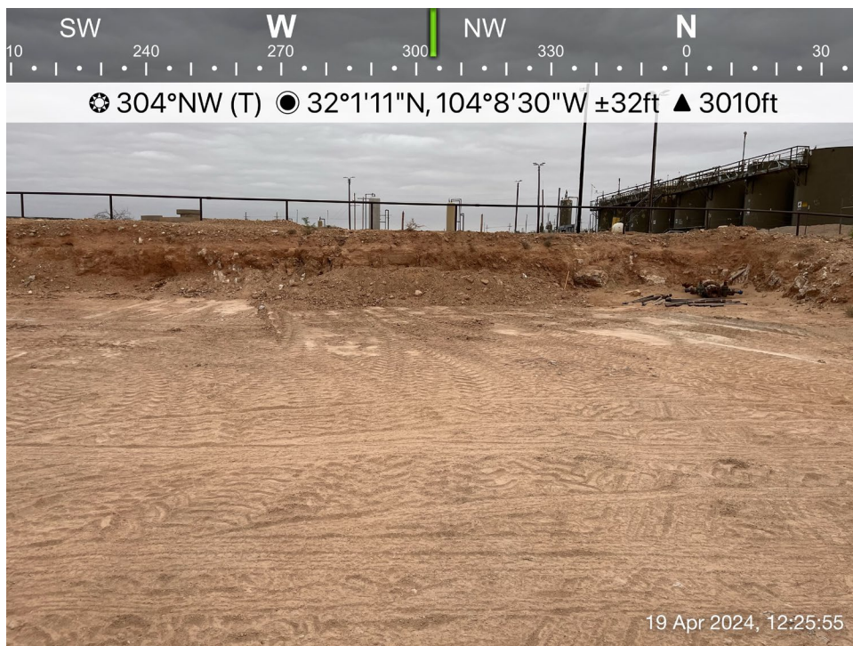
Backfilled excavation viewing northwest, April 15, 2024
