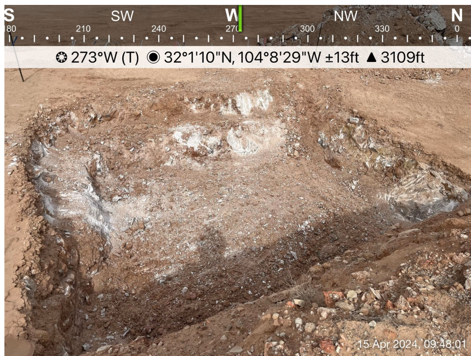
Excavated area encompassing S-9 to a depth of 6 feet viewing west, April 15, 2024
