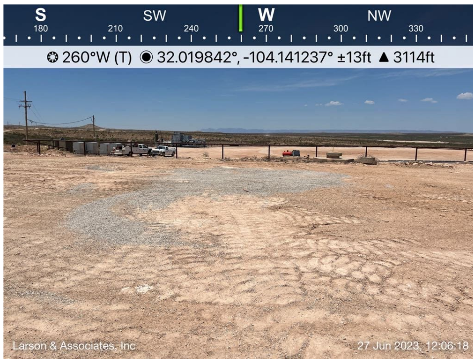
Impacted area viewing west, June 27, 2023
