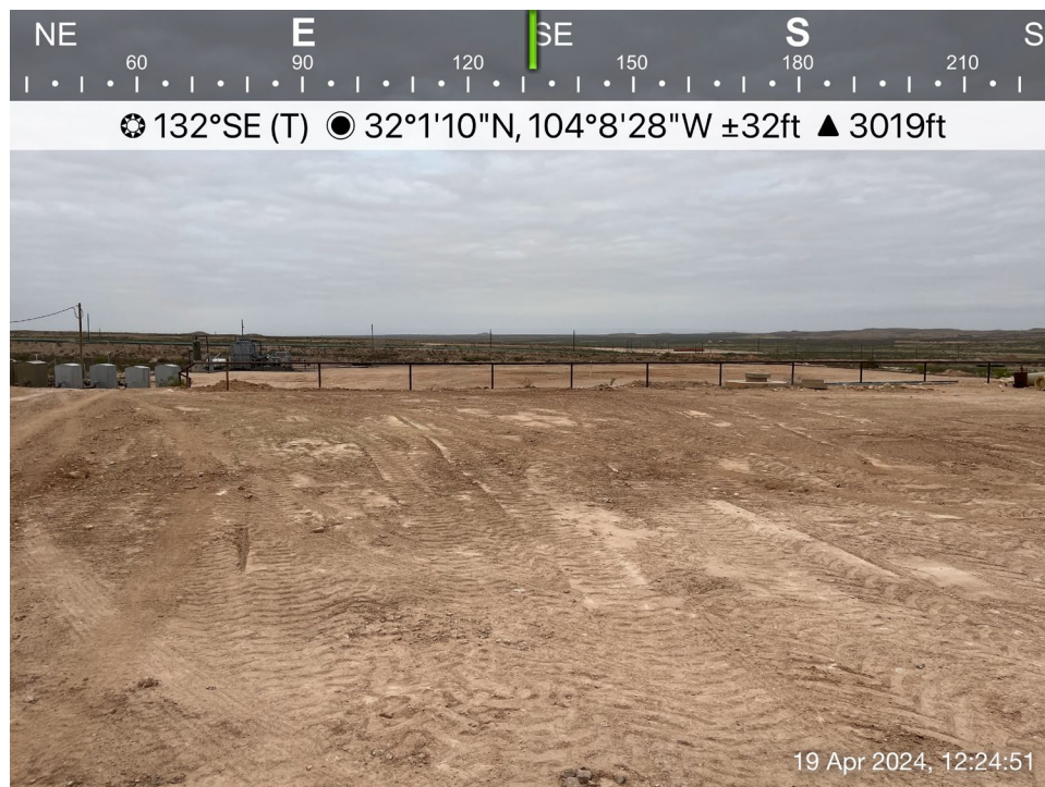
Backfilled excavation viewing southeast, April 19, 2024
