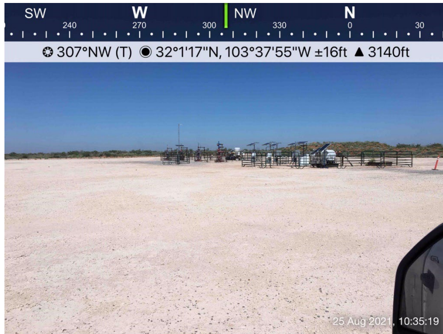
Impacted area on the pad, viewing to the northwest.
