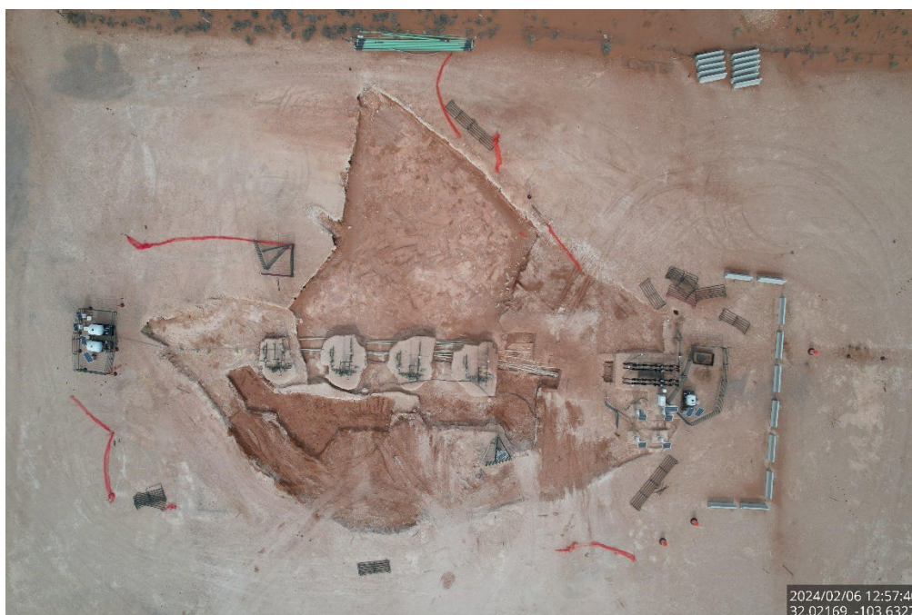
Aerial image of the excavation, vertical view.
