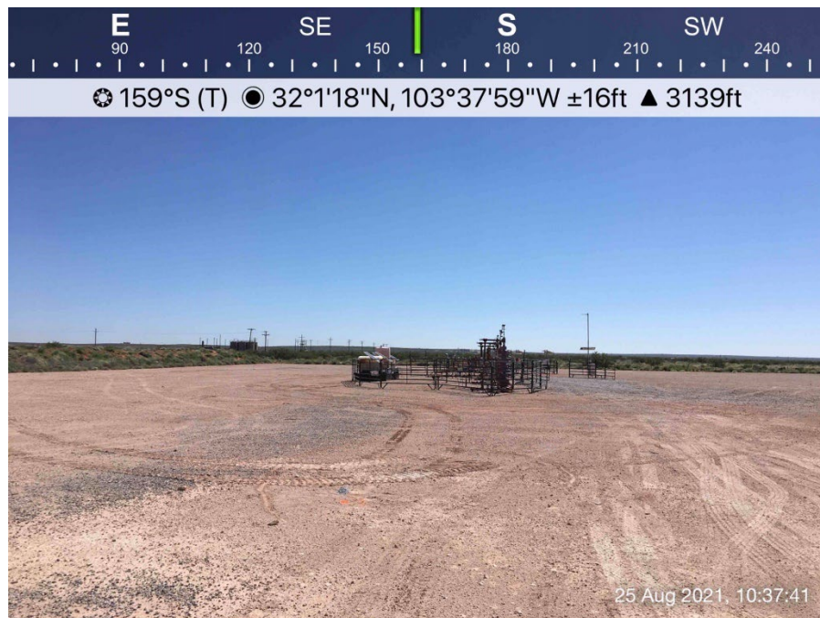
Impacted area on the pad, viewing to the south.
