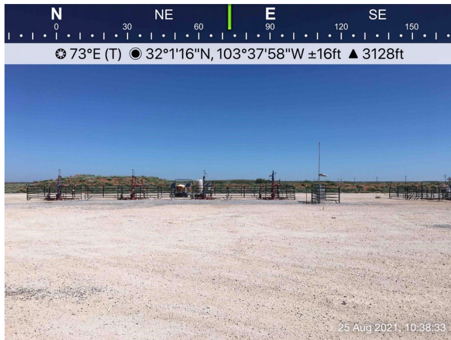
Impacted area on the pad, viewing to the north.
