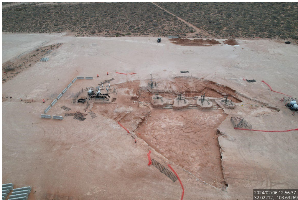
Aerial image of the excavation, viewing to the south.
