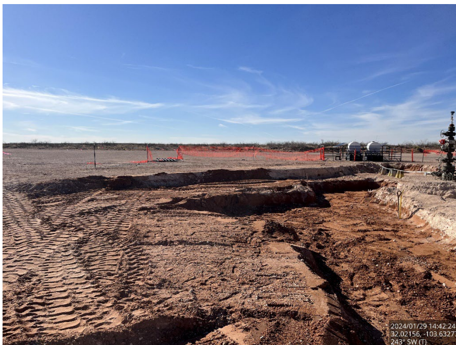
Excavated area on the pad, viewing to southwest.
