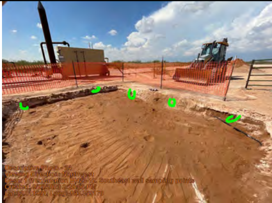
1 ft excavation BH23-12. Southeast wall sampling points
