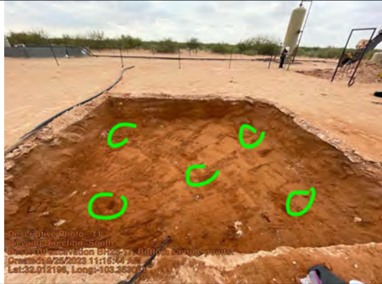
3ft excavation BH23-17. Bottom sample points.
