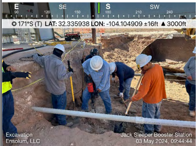
Photograph 15 Description: Excavation - Jack hammer rock View: South
