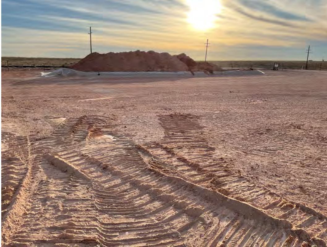
Excavated soil stockpile temporarily stored on plastic in contained area
