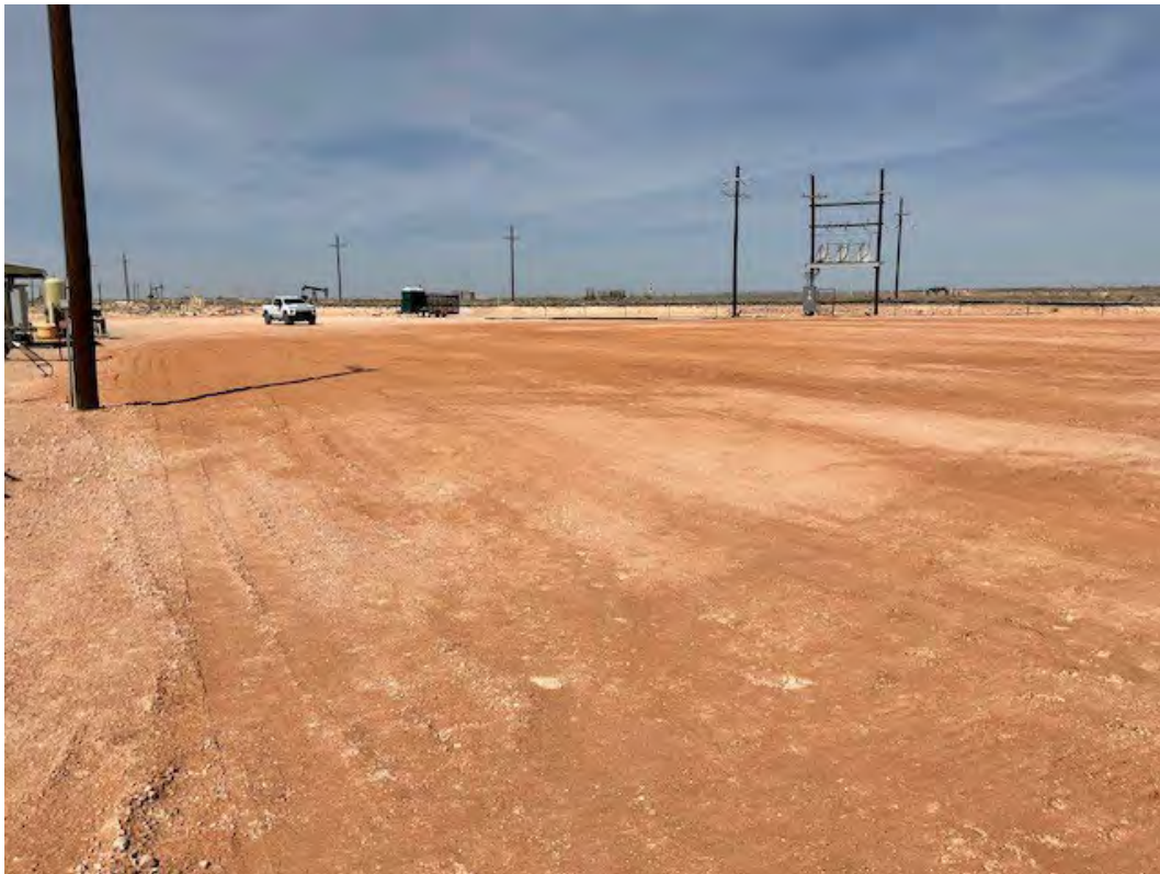
View north at backfilled and compacted area – on-site active pad
