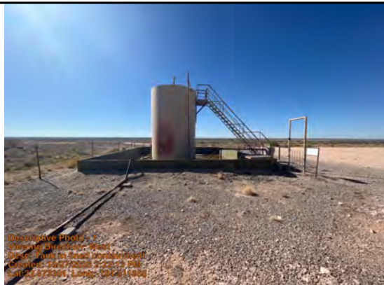
Tank in lined containment
