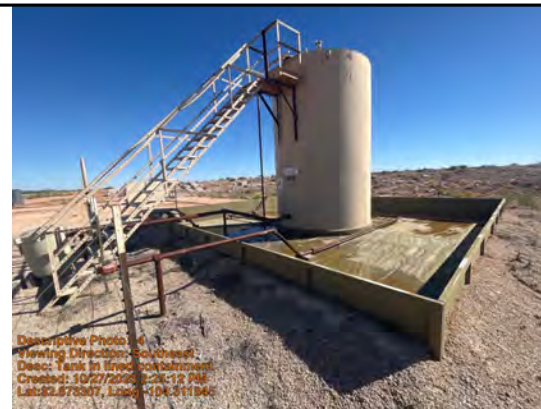
Tank in lined containment
