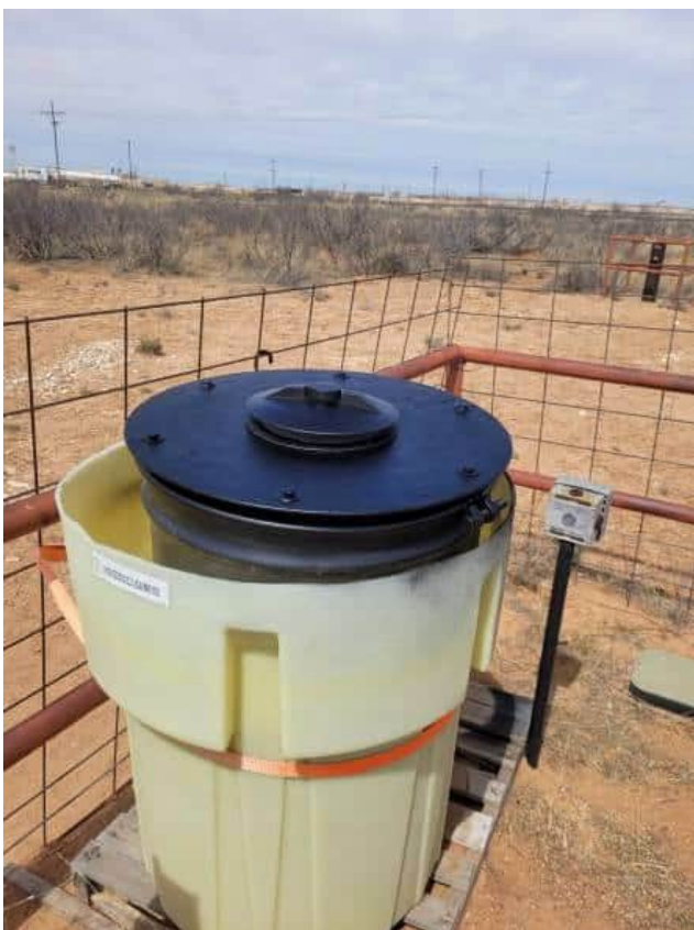
Jal #4 Gas Plant, Jal, New Mexico – IDW purgewater drum with WINDCRUSHER™ ventilated barrel cover successfully evaporates groundwater sampling Purgewater “24-7”, since 2020.
