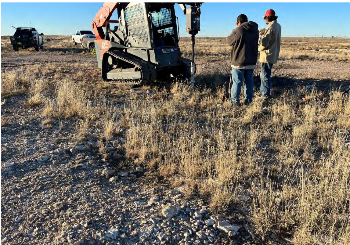
SP 2 – View north from a “background” boring C4. The Shahara pipeline is in the foreground and the spill footprint lies behind the auger rig (sun of January 3, 2024). The raised fill from the pipelines controls the shape of the release footprint.
