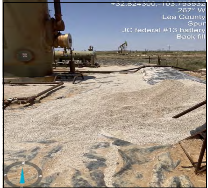
Photo showing backfill areas with clean gravel
