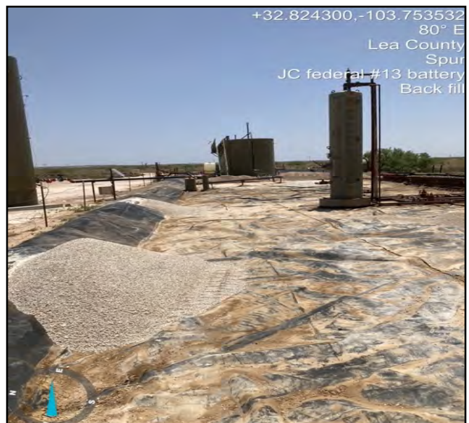
Photo showing backfill areas with clean gravel
