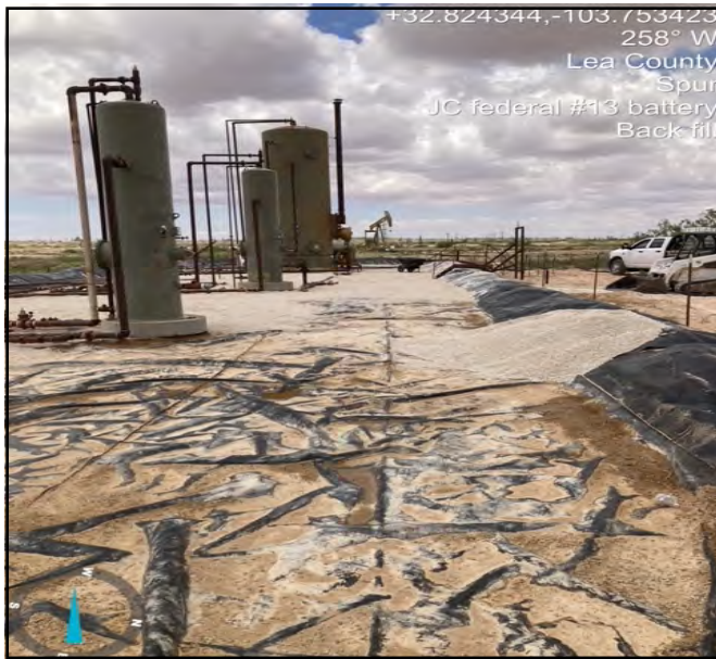
Photo showing backfill areas with clean gravel
