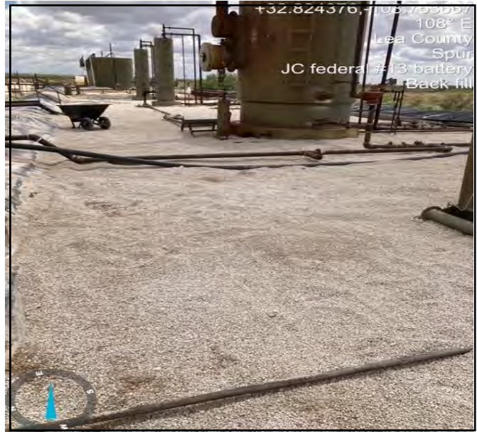
Photo showing backfill areas with clean gravel
