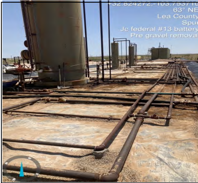
Photo exposing the liner that was underneath the contaminated gravel
