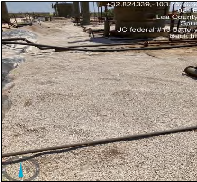
Photo showing backfill areas with clean gravel
