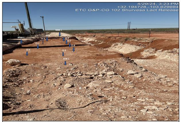
View North - Remediation activites (i.e., excavation and stockpiling) and sampling CS 1 thru CS 9, WSW 1, NSW 1 and SSW 1 in progress.
