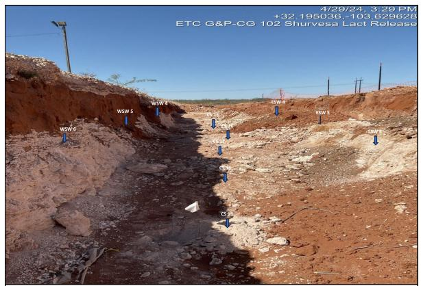
View North - Remediation activites (i.e., excavation and stockpiling) and sampling CS 15 thru CS 19, WSW 4 thru WSW 6 and ESW 4 thru ESW 6 in progress.
