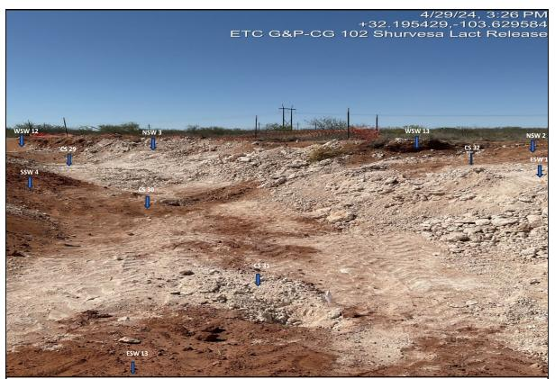
View West - Remediation activites (i.e., excavation and stockpiling) and sampling CS 29 thru CS 32, WSW 12, WSW 13, NSW 2, NSW 3, ESW 12, ESW 13 Date: Apr 29, 2024 and SSW 4 in progress.
