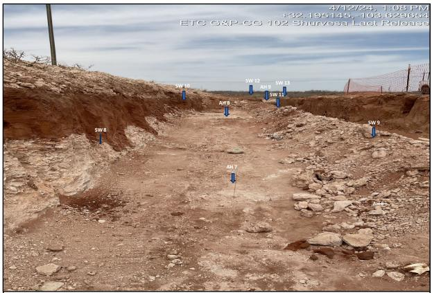
View North - Remediation activites (i.e., excavation and stockpiling) and sampling of AH 7 thru AH 9 and SW 8 thru SW 13 in progress.
