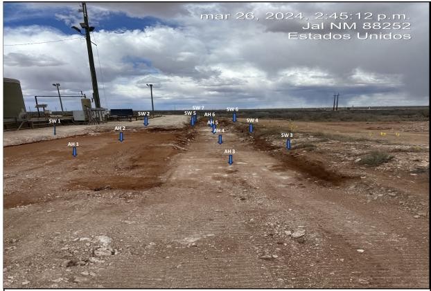
View North - Remediation activites (i.e., excavation and stockpiling) and sampling of AH 1 thru AH 6 and SW 1 thru SW 7 in progress.
