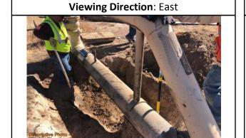
Hand dug excavation under pipe at point of release
