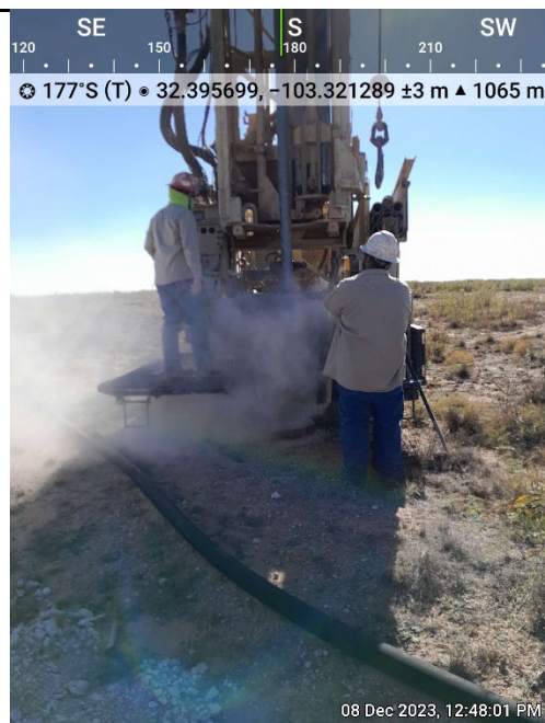
Photograph 4 Date: 12-8-2023 Description: Delineation activities-air rotary View: South
