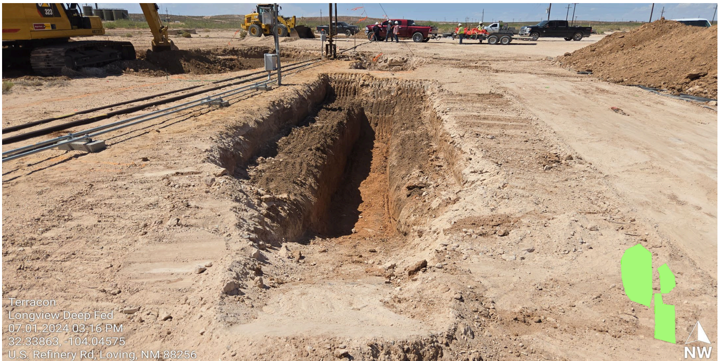
Photo 6 Completed excavation around southern extent 6' bgs
