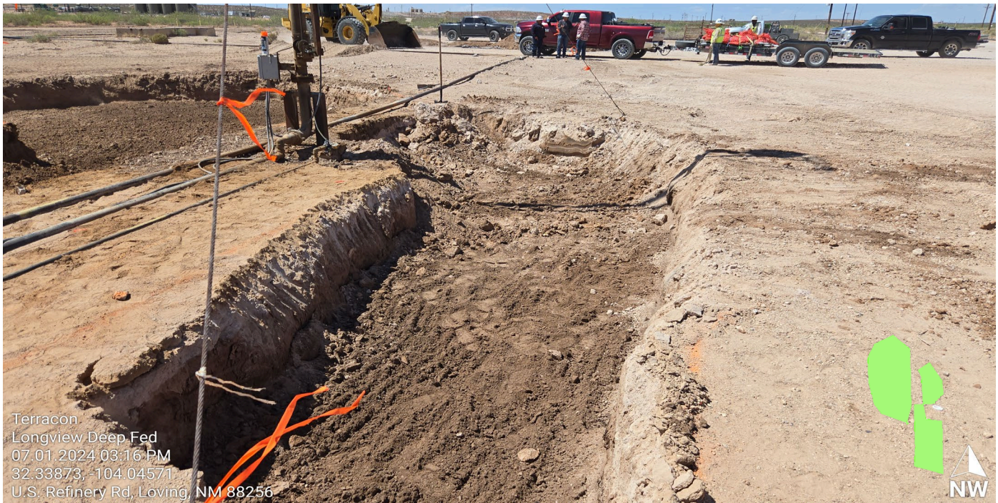
Photo 5 Completed excavation around northeastern extent 2' bgs
