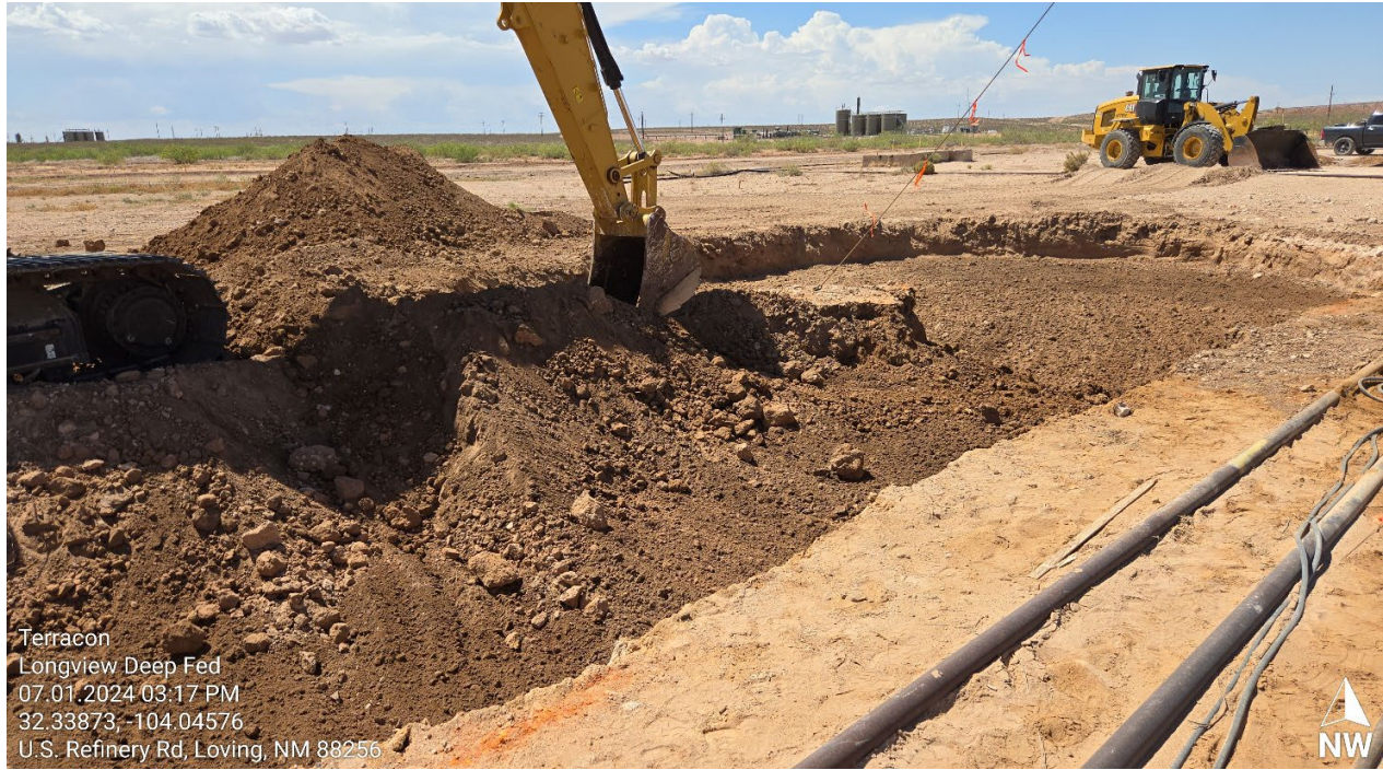
Photo 7 Excavation in progress around northwestern extent 2-6' bgs
