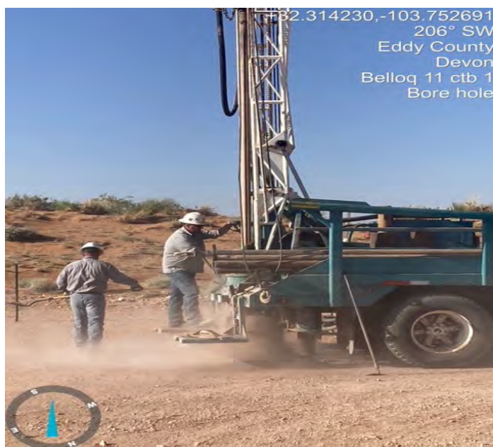
Drilling borehole to 105'
