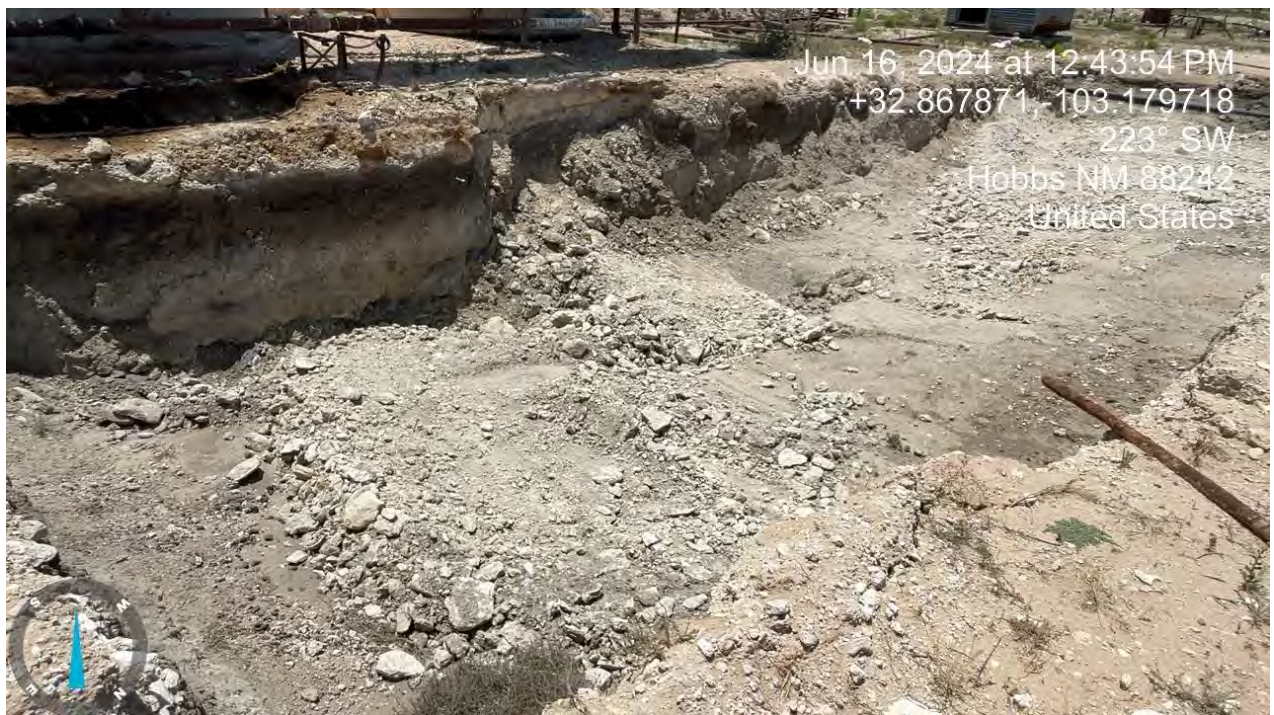
South sidewall showing length of hydrocarbon impacts, existing infrastructure prevents further excavation
