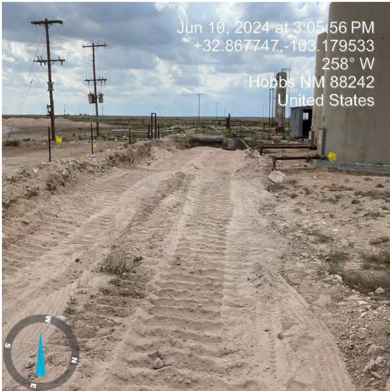
South excavation compacted backfill prepared for drilling of boreholes #1 and #2
