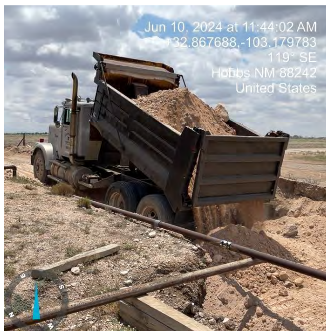
Preparing south excavation for borehole drilling with clean caliche backfill
