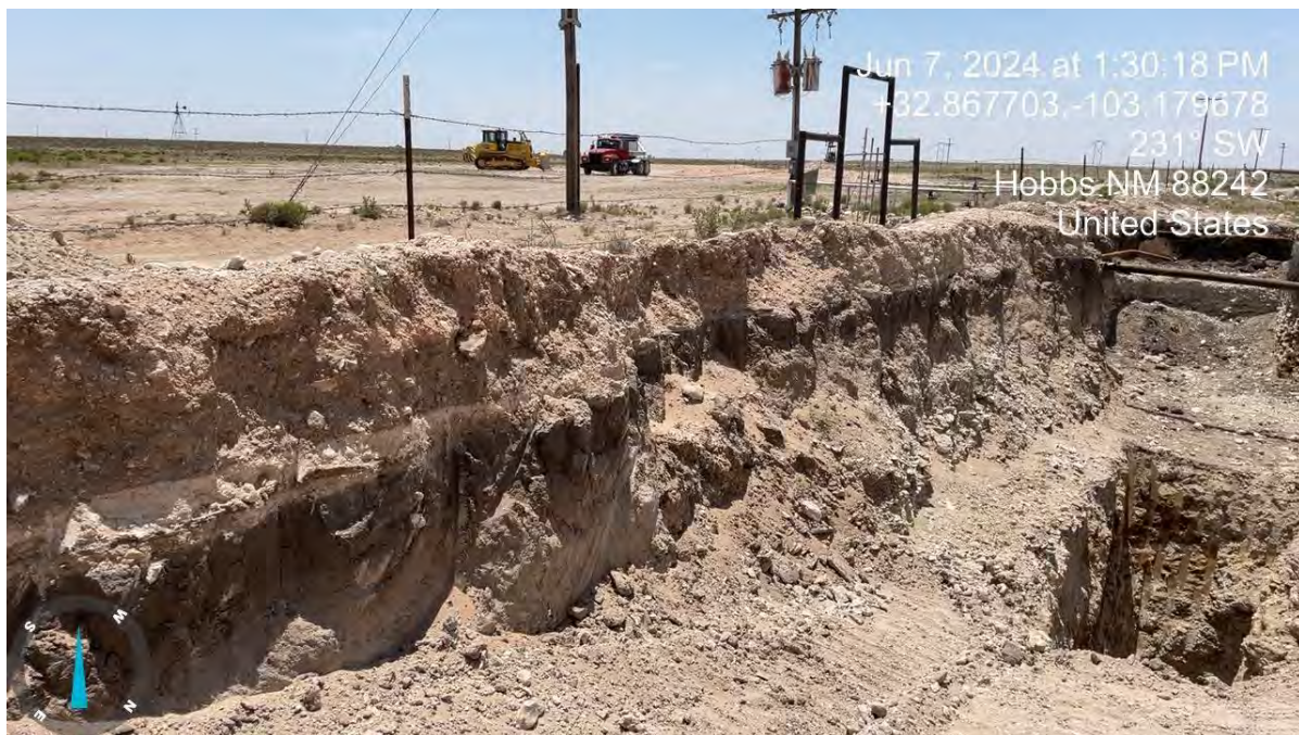
South berm wall showing hydrocarbon impacts, delineation excavation at right
