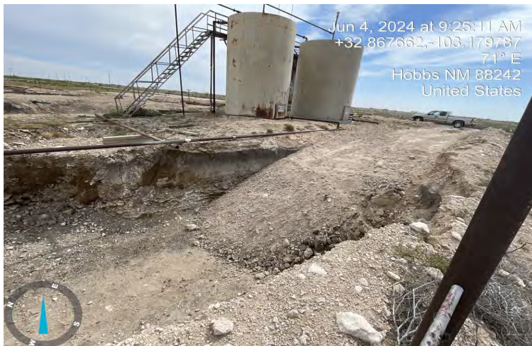
View looking northeast, hydrocarbon impacts north of flow line not accessible for excavation
