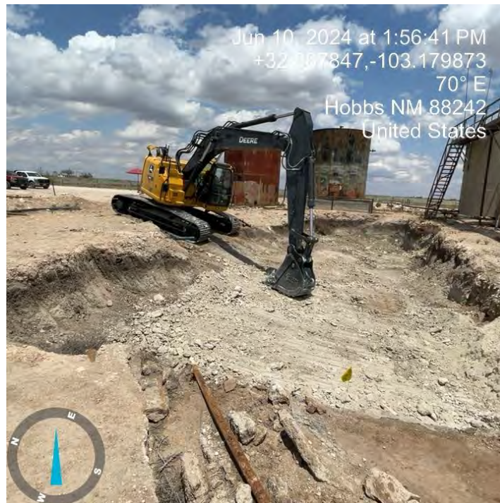
Trackhoe preparing north excavation for drilling
