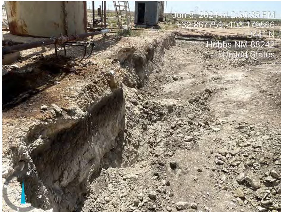
South sidewall in vicinity of sample location N-3 showing hydrocarbon impacts
