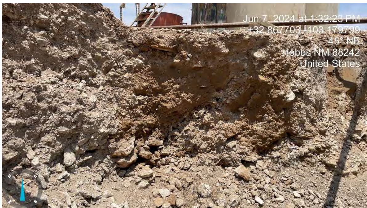
Hydrocarbon impacts vicinity of sample location S-3. Infrastructure prevents further excavation
