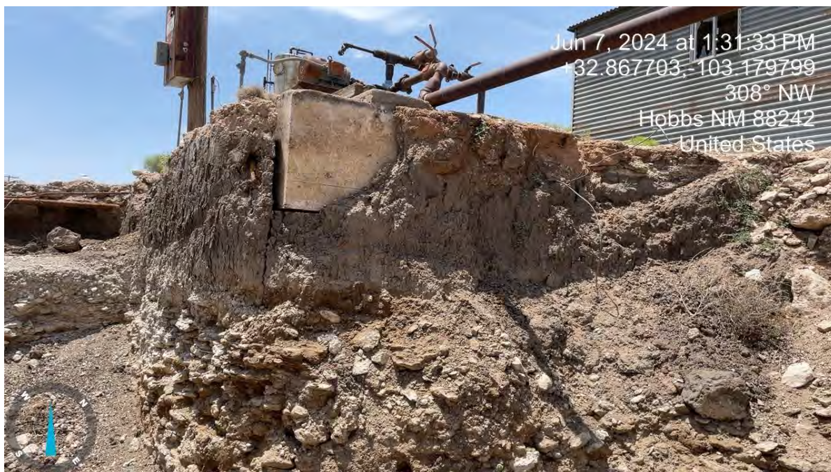
Northwest corner of trench showing hydrocarbon impacts below transfer pump and concrete pad
