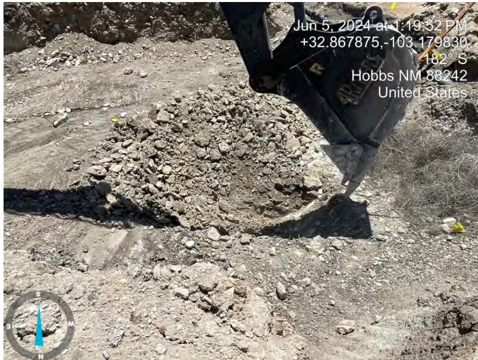
Unsuccessful attempt of vertical delineation vicinity of sample location N-8, Borehole #4 was drilled at this location
