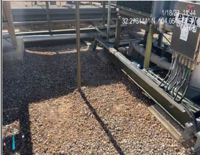
Photograph 1 Date: 01/18/2023 Description: Southern view of initial Site assessment activities
