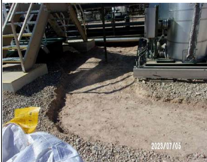
Photograph 4 Date: 07/05/2023 Description: Western view of restoration activities
