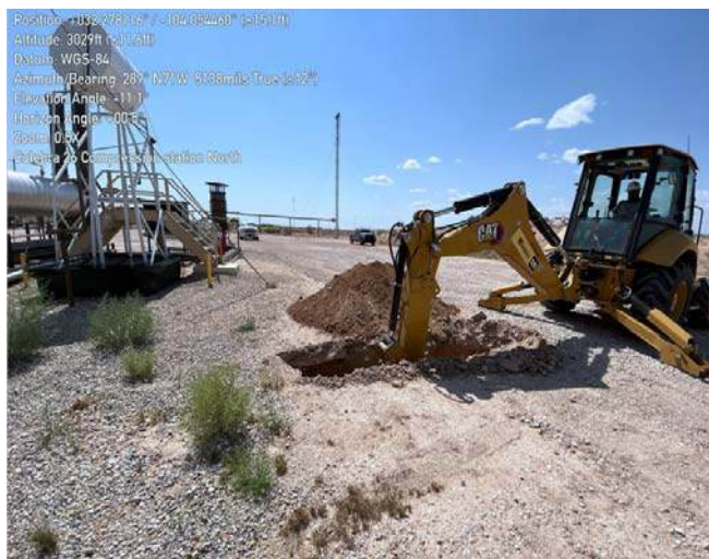
Photograph 8 Date: 07/17/2024 Description: Northwestern view of Delineation activities
