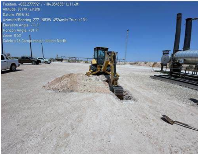
Photograph 1 Date: 07/17/2024 Description: Northwestern view of Delineation activities
