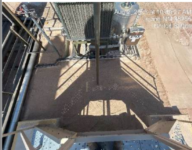
Photograph 7 Date: 08/02/2023 Description: Aerial view of restoration activities
