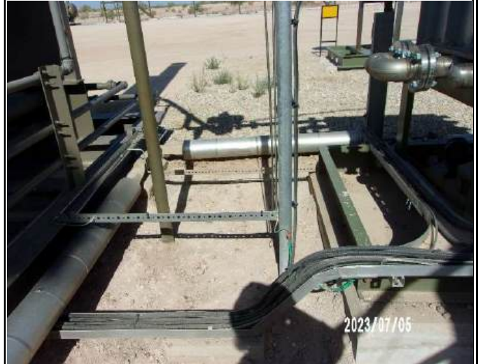
Photograph 6 Date: 07/05/2023 Description: Southern view of excavation activities
