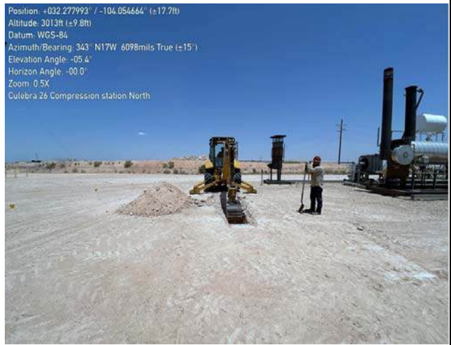
Photograph 2 Date: 07/17/2024 Description: Northwestern view of Delineation activities
