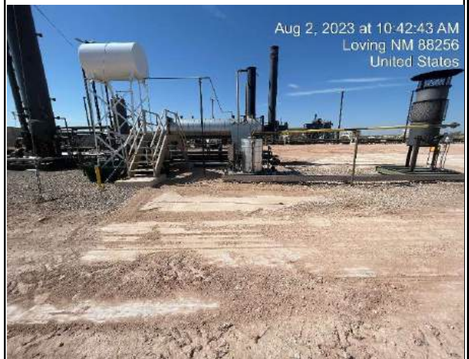
Photograph 8 Date: 08/02/2023 Description: Southern view of restoration activities
