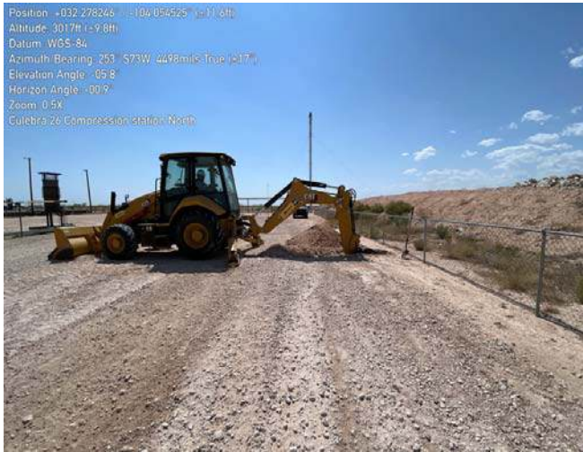
Photograph 5 Date: 07/17/2024 Description: Southwestern view of Delineation activities
