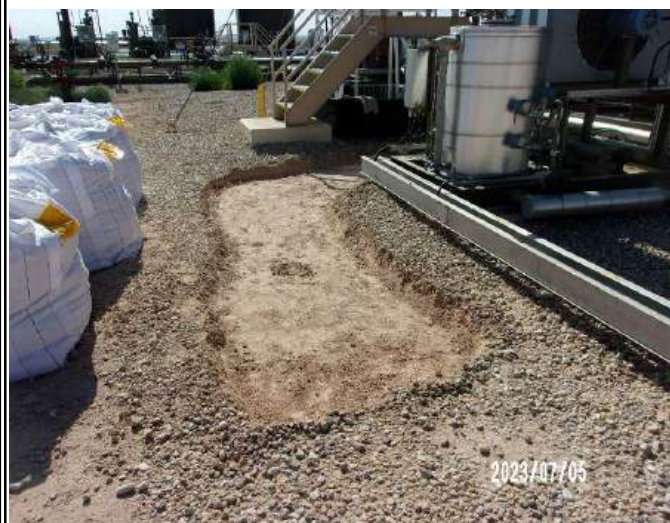
Photograph 3 Date: 07/05/2023 Description: Western view of excavation activities
