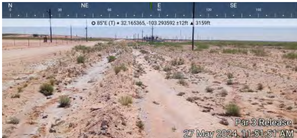
Figure 1: Eastern release extent that flowed along a pipeline ROW containing seven pressurized flowlines.
