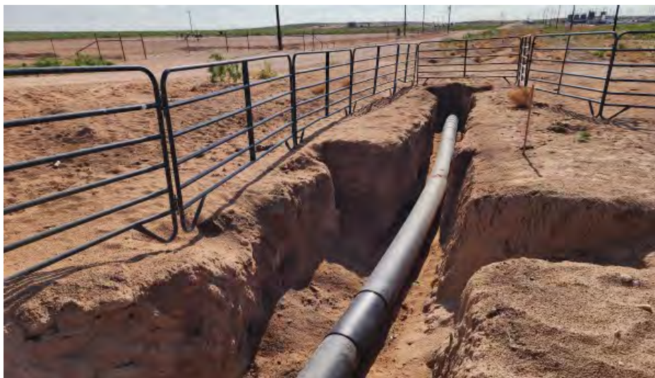
Figure 2: Excavation area during flowline repair. Viewing east from near the source. 06/10/2024. 32.1653333 N, 103.2939297 W
