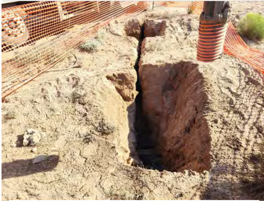
Figure 3: Hydrovac windows for line spotting and soil sampling near CS-09. 07/19/2024. 32.1653289 N, 103.2922439 W
