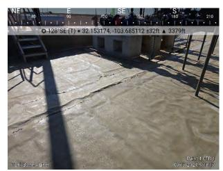
Photograph 15 Date: 9/17/24 Description: Separator Containment Liner
