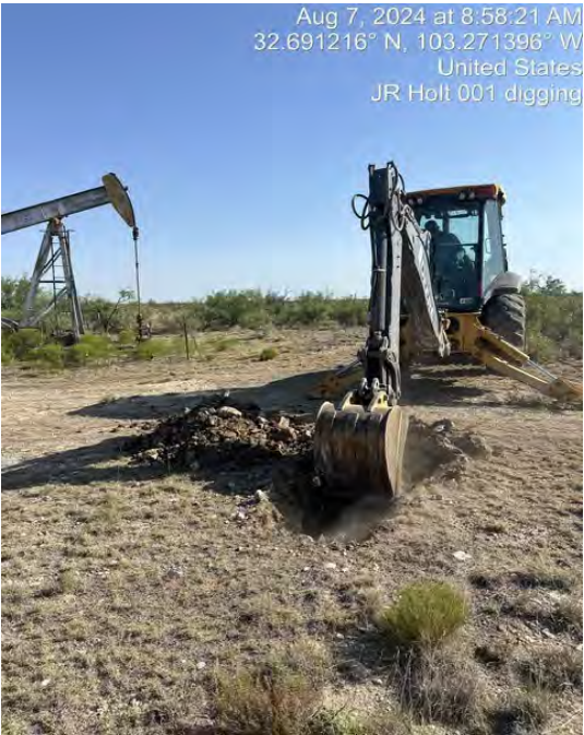
View to E of Sample 1 location (8/7/24).
