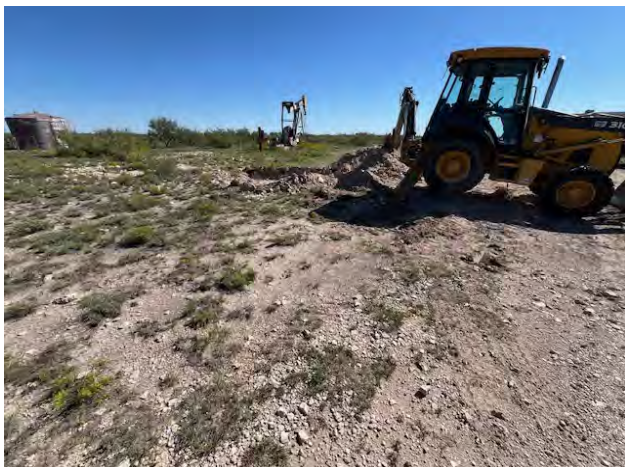
View to E of excavating (9/25/24).
