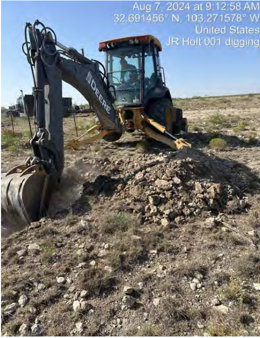
View of test hole sampling (8/7/24).
