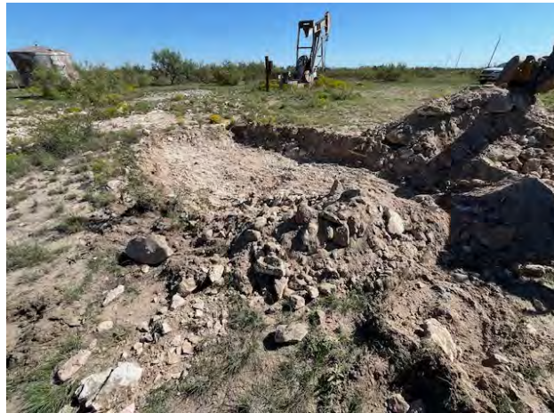
View to NE of excavation (9/25/24).
