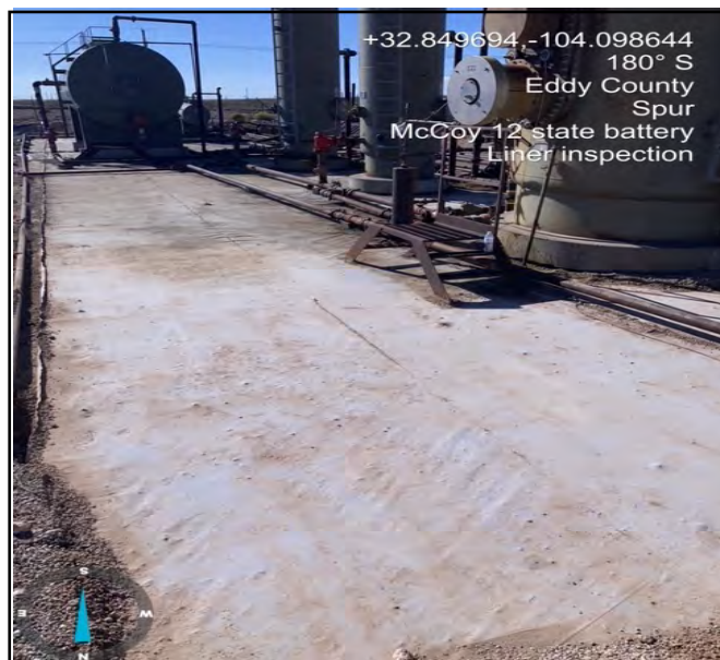
Photo of liner being inspected facing South.
