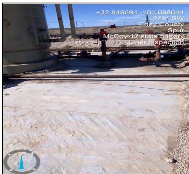
Photo of liner being inspected facing Southwest.
