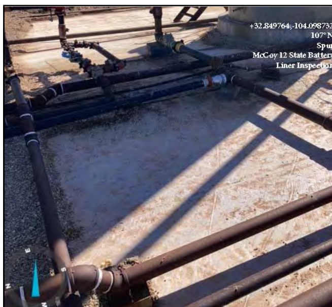
Photo of liner being inspected facing North.
