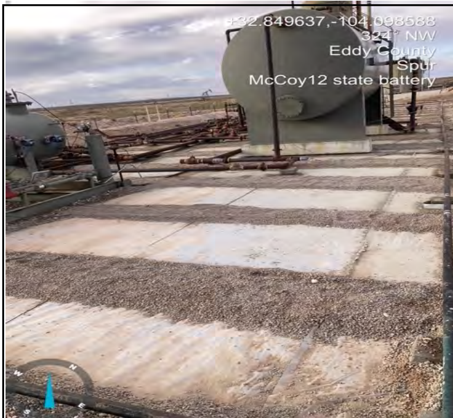
Photo of liner being backfilled with clean material to form wind rows facing Northwest.
