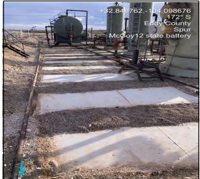
Photo of liner being backfilled with clean material to form wind rows facing South.
