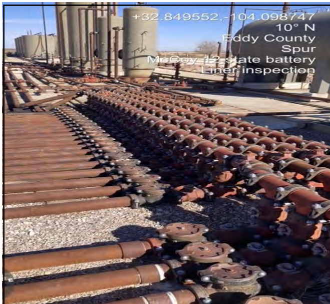
Photo of liner being inspected facing North.
