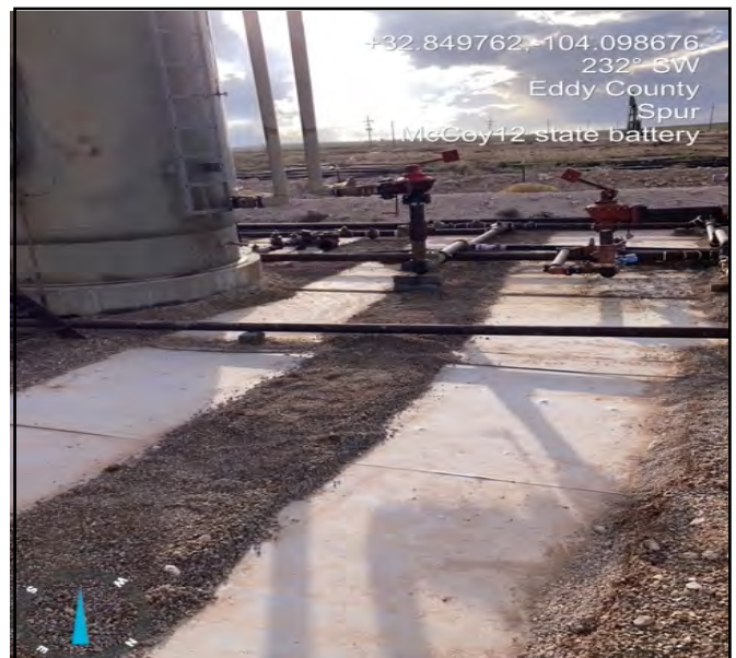
Photo of liner being backfilled with clean material to form wind rows facing Southwest.
