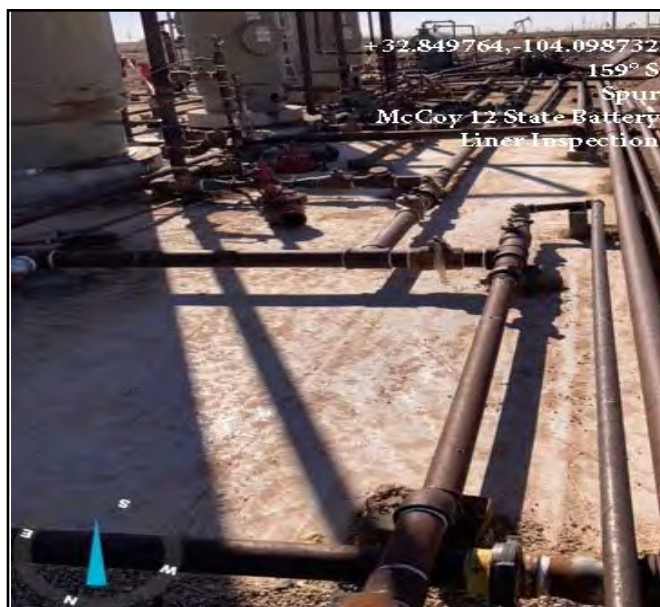
Photo of liner being inspected facing South.
