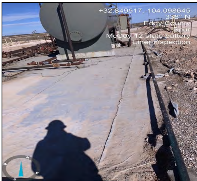
Photo of liner being inspected facing North.
