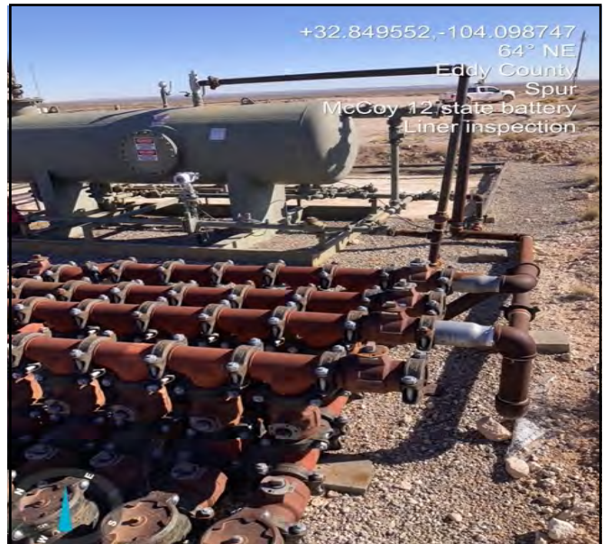
Photo of liner being inspected facing Northeast.
