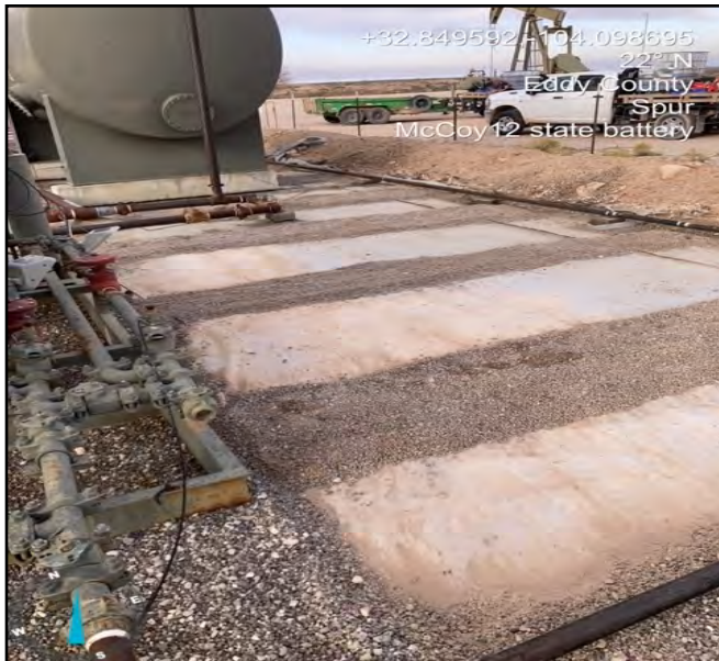
Photo of liner being backfilled with clean material to form wind rows facing North.
