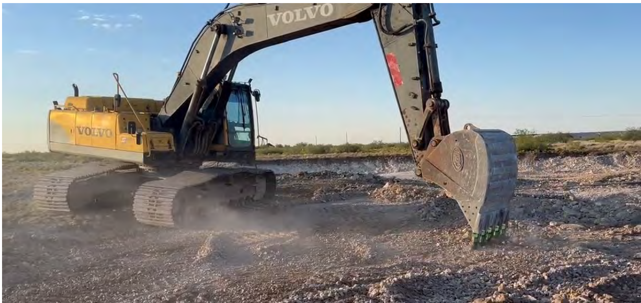
Figure 3: Trackhoe with Sharks Teeth attempting to break through the hard caliche in the 1 to 2 foot area. October 11, 2024.
