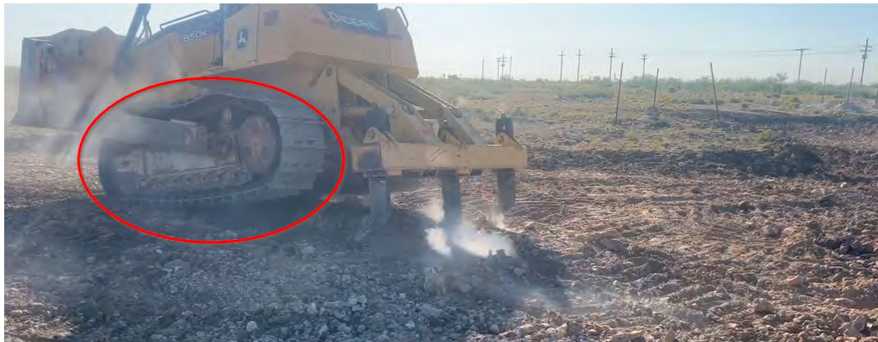
Figure 1: Rippers on the bulldozer could not breakup the hard caliche. The rear of the dozer was lifted (circled red) by putting all the pressure on the rippers. October 10, 2024.
