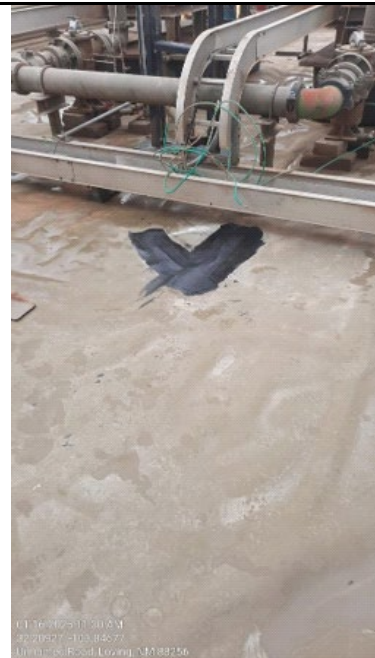
Photograph: 4 Date: 1/16/2025 Description: Liner Patch View: Direct
