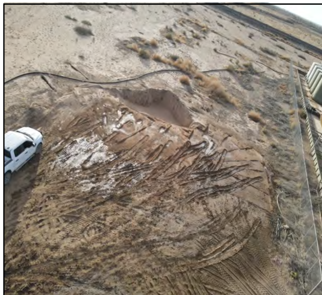
Photo of the release area being backfilled.
