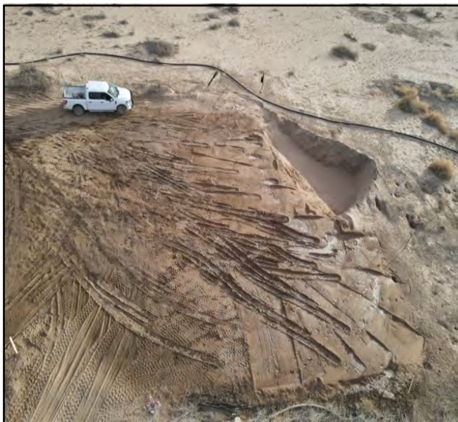
Photo of the release area being backfilled.
