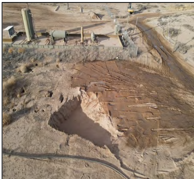
Photo of the release area being backfilled.
