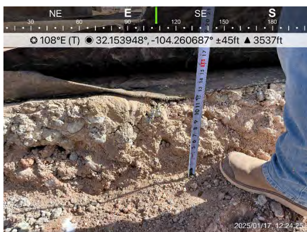
Figure 11. Excavation depth verification.
