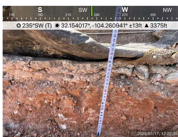
Figure 12. Excavation depth verification.
