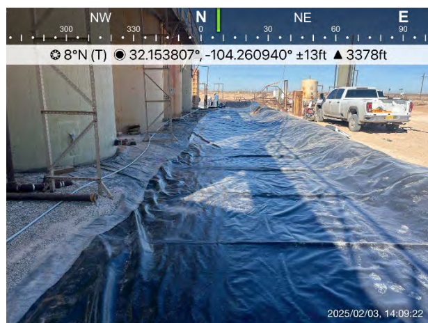
Fig. 35. Liner repaired at the 5-foot buffer mark.
