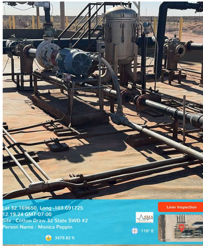
Photograph #10: Liner under sandpot filter and transfer pump.
