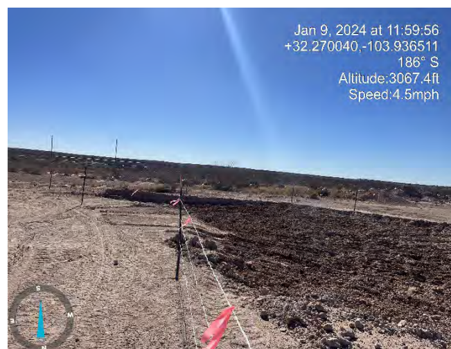
Photograph 3 Date: 01/09/2024 Description: Excavation activities View: South
