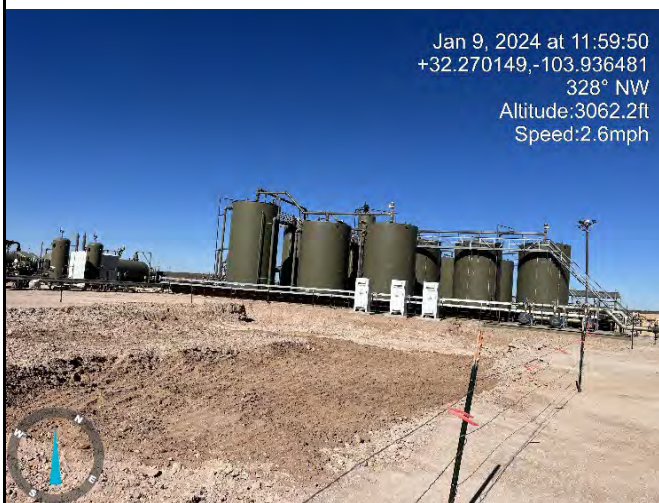
Photograph 2 Date: 01/09/2024 Description: Excavation activities View: Northwest
