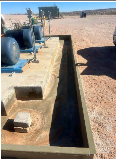
Photograph 3 Date: 01/13/2023 Description: Liner inspection activities. View: East
