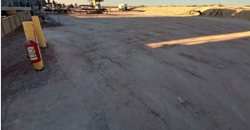
PHOTO 12: Southwestern view during restoration activities. 10/11/2024
