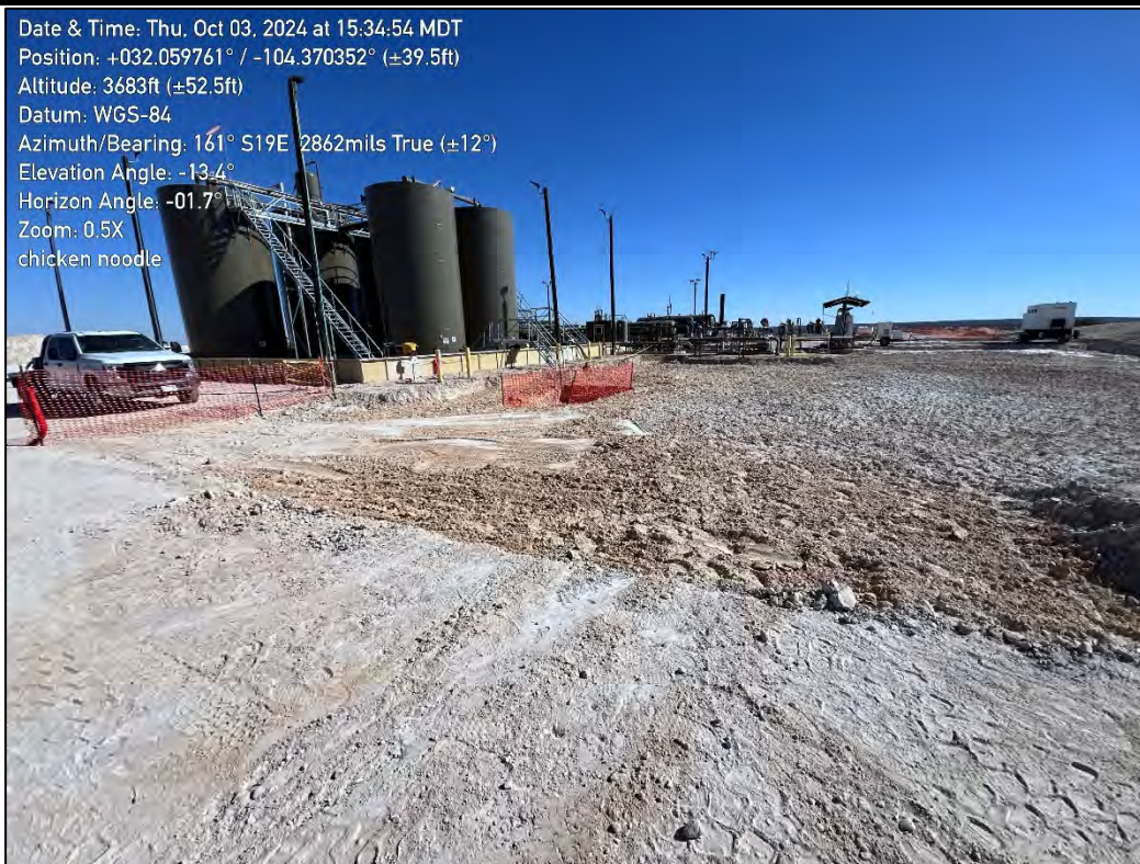
PHOTO 7: Southeastern view of excavation extent. 10/03/2024
