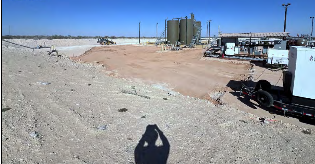
PHOTO 11: Northeastern view during restoration activities. 10/08/2024
