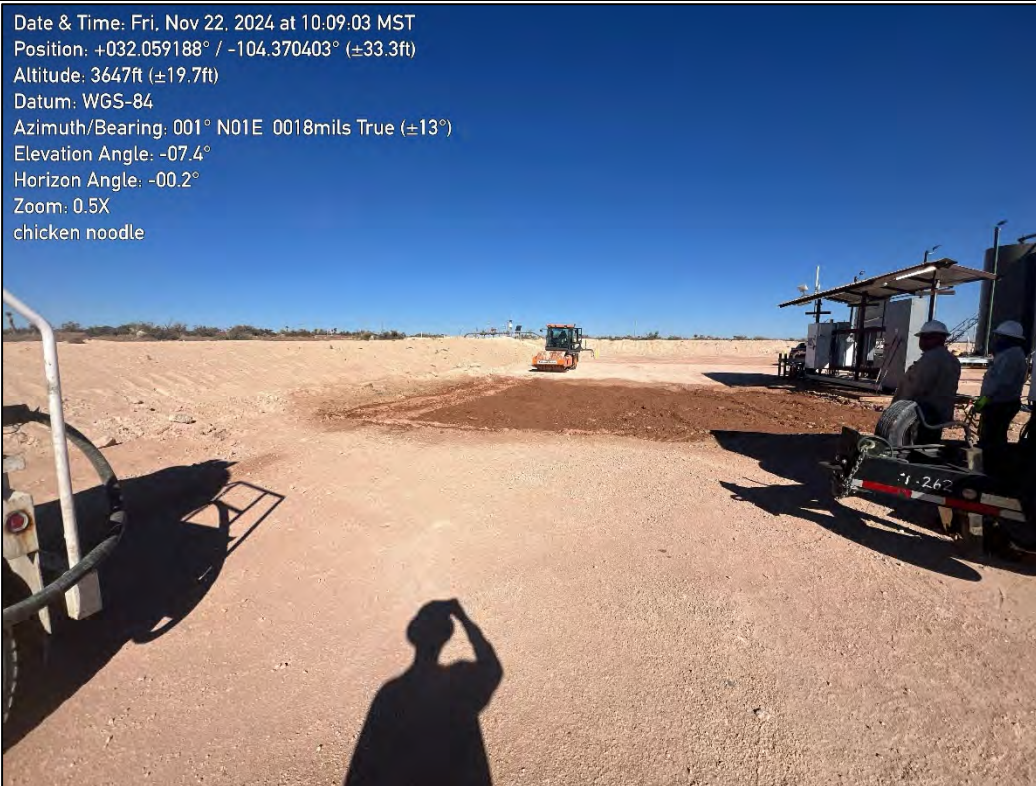
PHOTO 17: Northeastern view during continued restoration activities. 11/22/2024
