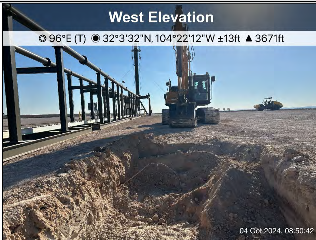
PHOTO 8: Northwestern view during excavation activities. 10/04/2024
