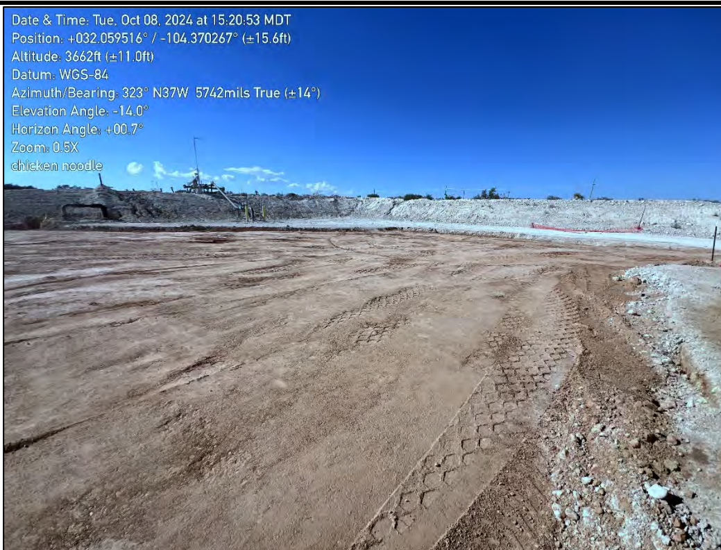
PHOTO 10: Northwestern view during restoration activities. 10/08/2024
