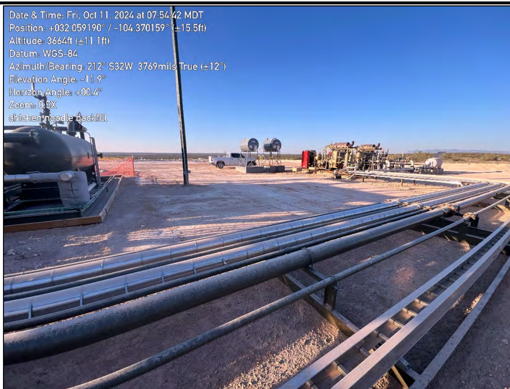
PHOTO 14: Southwestern view during restoration activities. 10/11/2024
