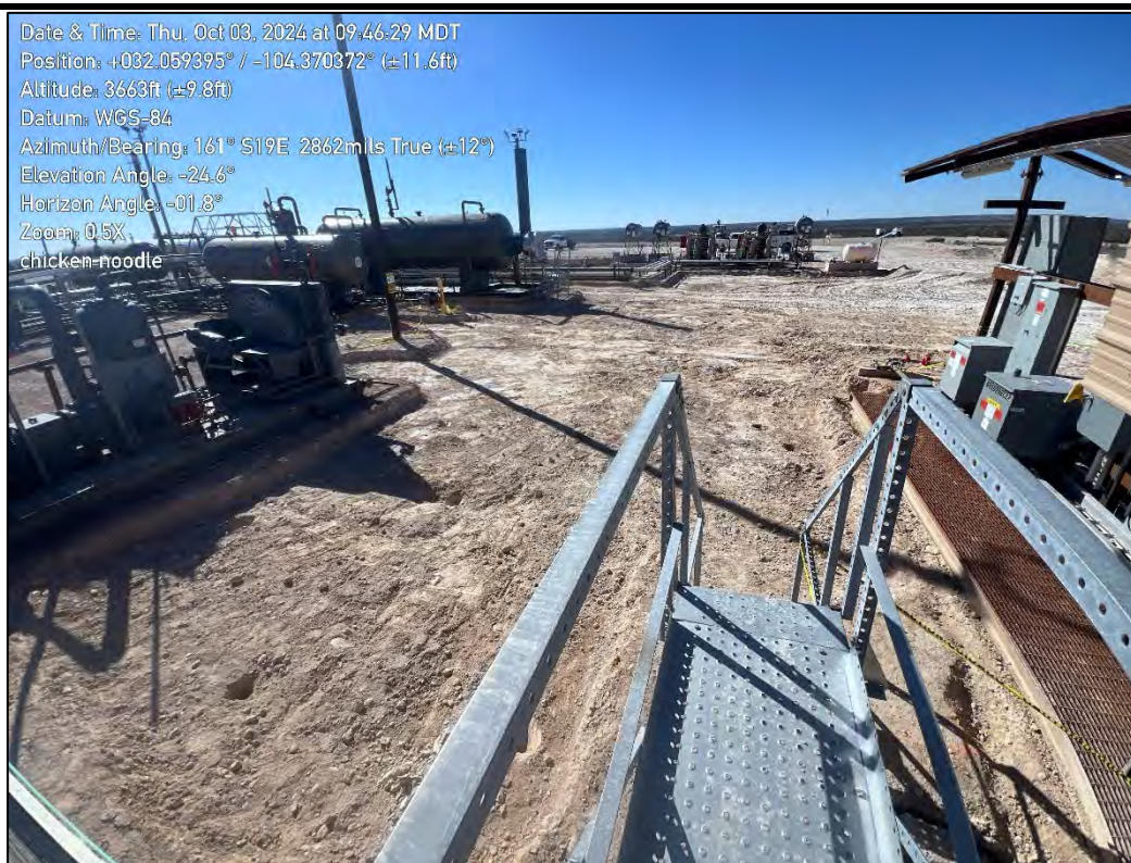
PHOTO 6: Southeastern view during excavation activities. 10/03/2024
