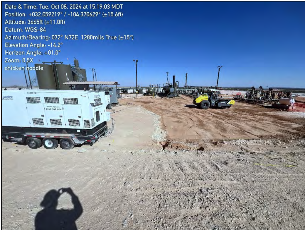
PHOTO 9: Northeastern view during restoration activities. 10/08/2024
