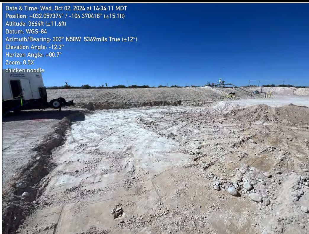
PHOTO 4: Northwestern view during excavation activities. 10/02/2024
