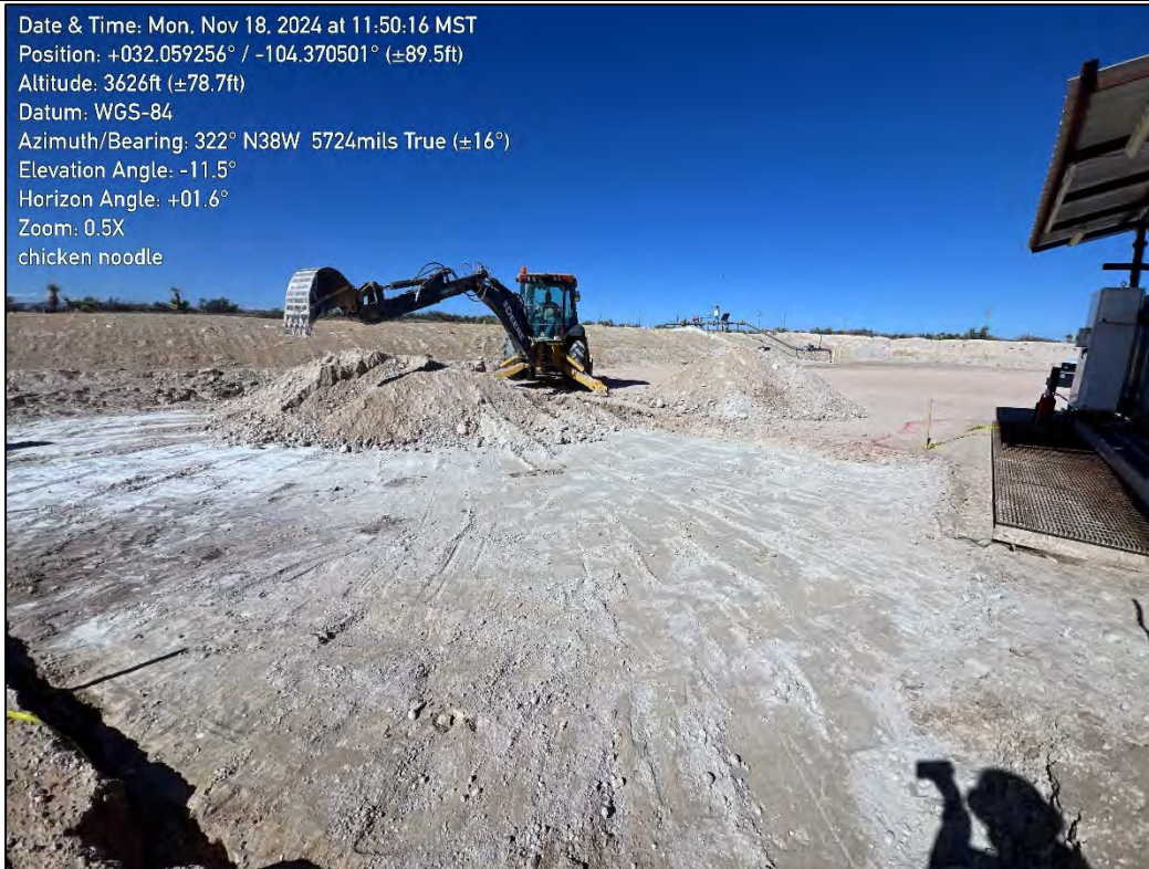
PHOTO 15: Northwestern view during continued excavation activities. 11/18/2024
