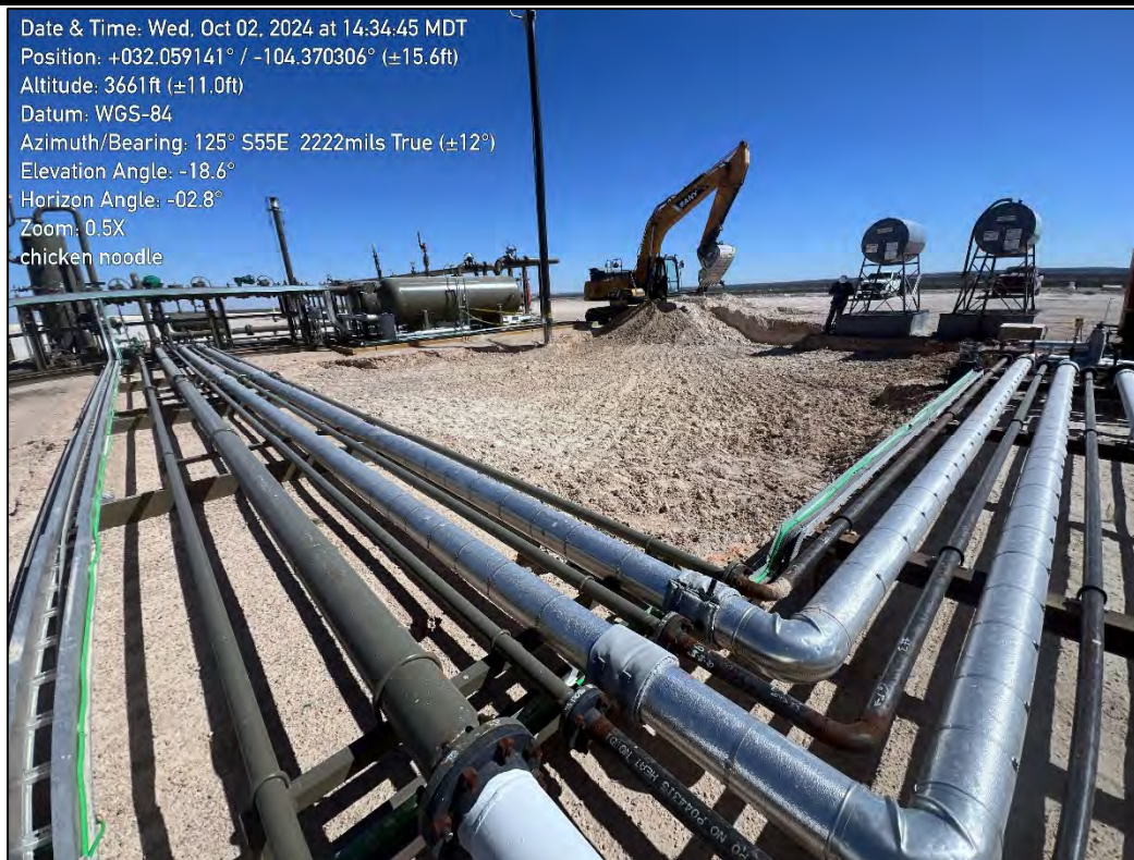
PHOTO 5: Southeastern view during excavation activities. 10/02/2024
