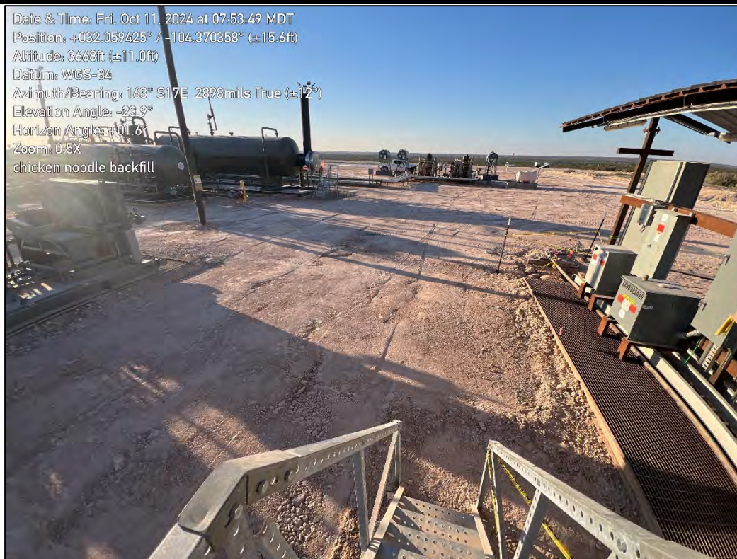
PHOTO 13: Northeastern view during restoration activities. 10/11/2024
