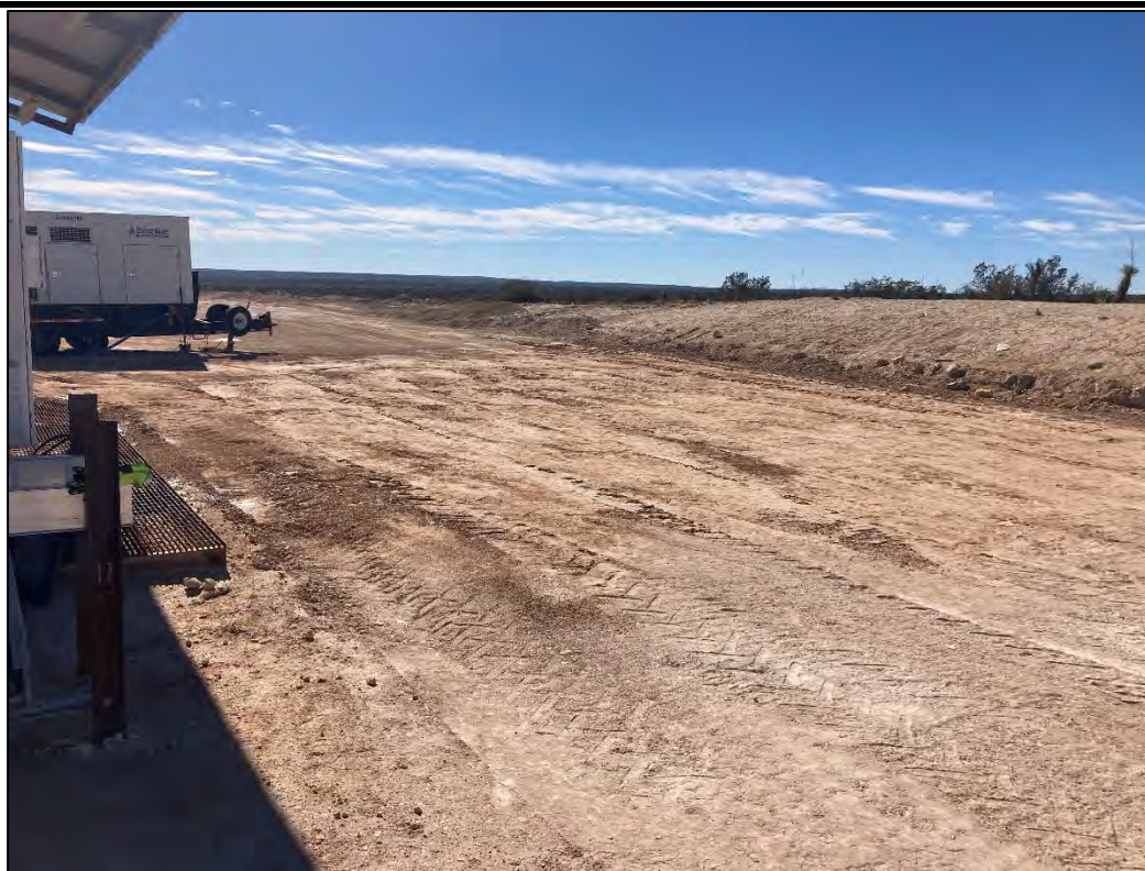
PHOTO 18: Southeastern view during restoration activities. 11/22/2024
