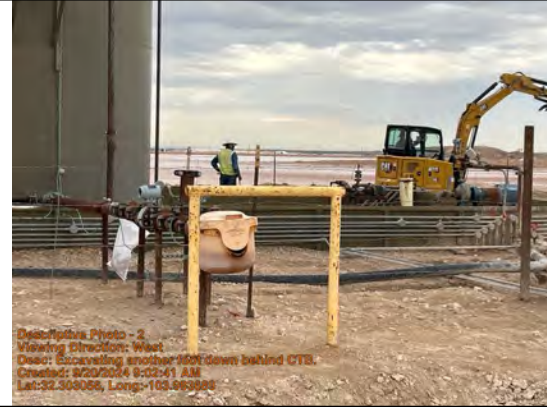
Excavating another foot down behind CTB.
