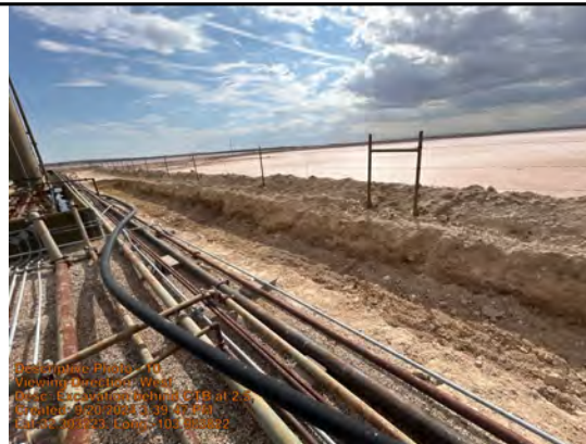
Excavation behind CTB at 2.5'
