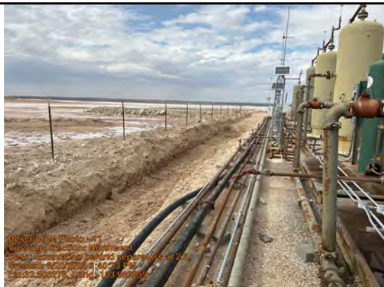
Excavation behind separators at 2.5'
