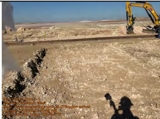
Crew excavating north of CTB upon arrival
