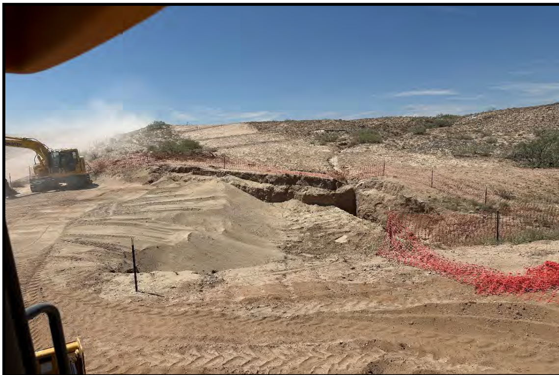
View of the excavation activities
