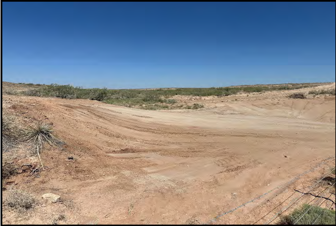
View of the backfilled area.
