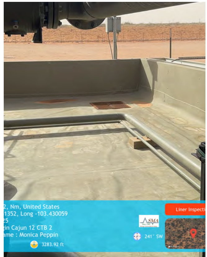
Photograph #14: Facing south viewing southwest corner.
