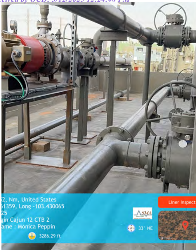
Photograph #11: Northwest area of containment.
