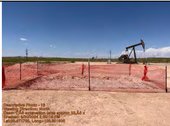
1' excavation (size approx 23' x 16')
