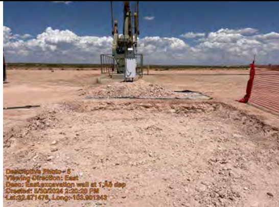
East excavation wall at 1' depth
