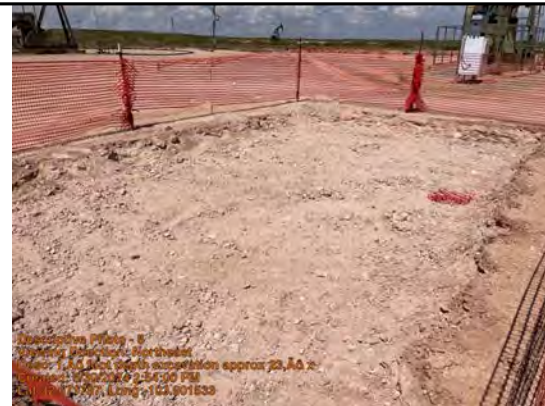
Southwest corner of 1' foot depth excavation facing the northeast (excavation size approx 23' x 16') approx 23' x 16'
