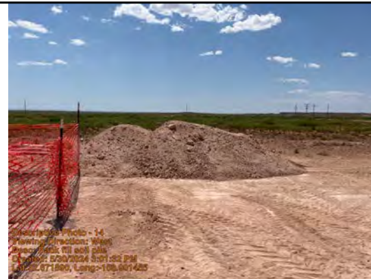
Back fill soil pile
