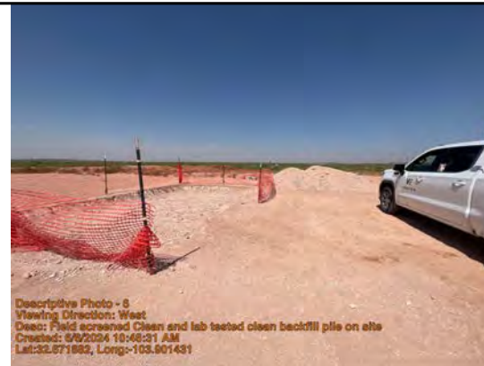
Field screened Clean and lab tested clean backfill pile on site
