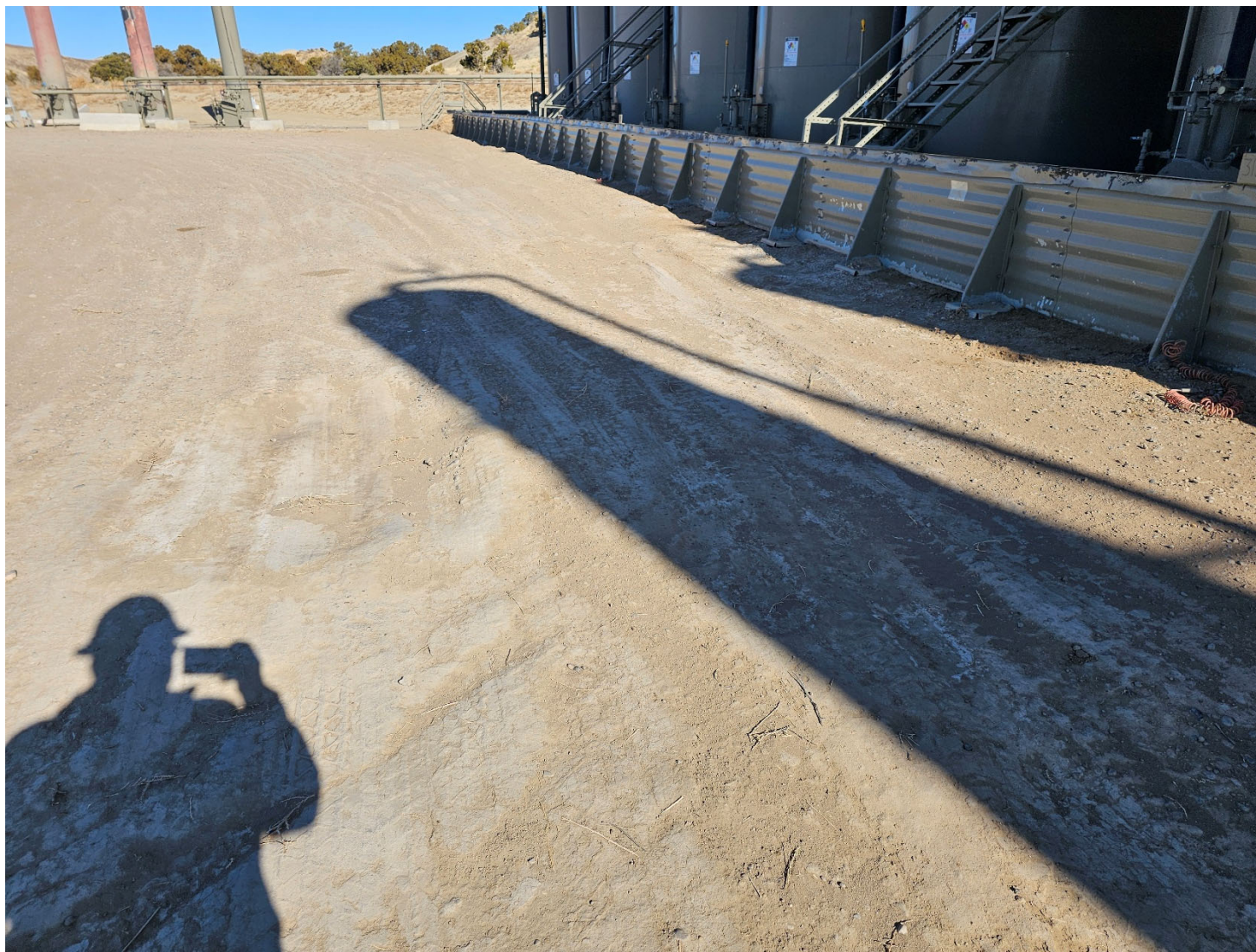
Photo #2 Additional area outside of containment.
