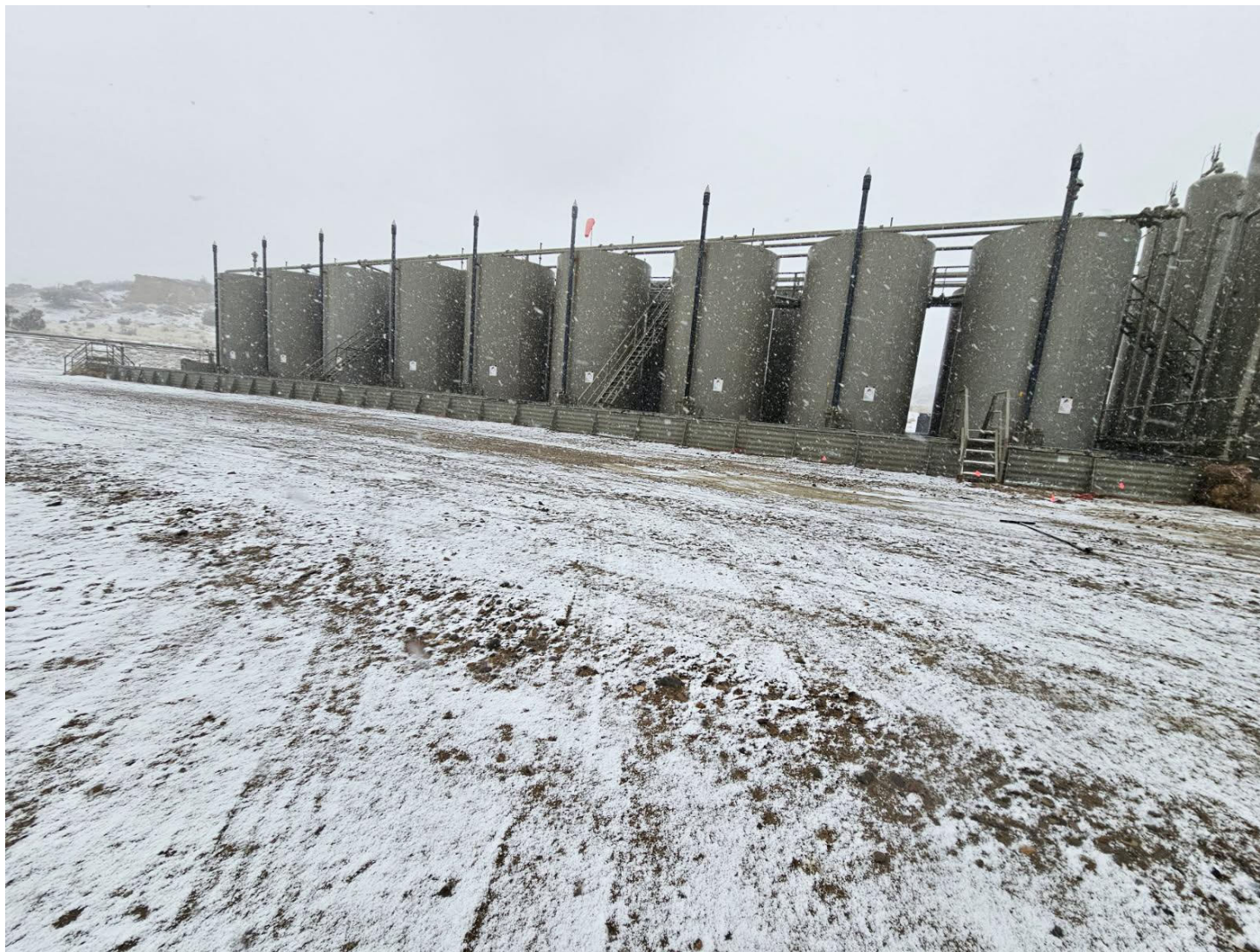
Photo #3 Post-excavation soil sampling outside containment area.
