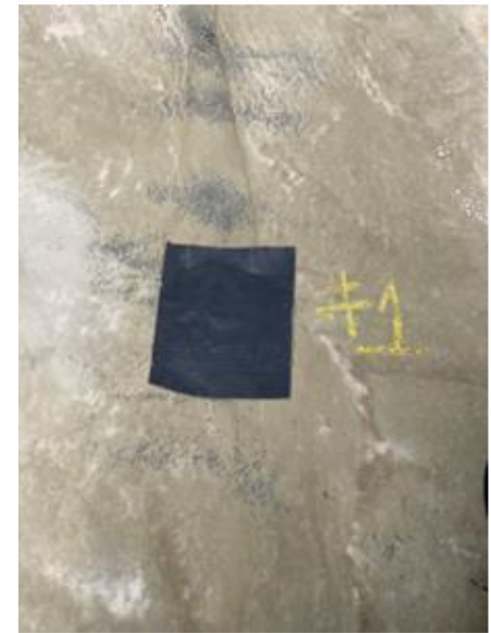
Liner Sample Point #1-patched
