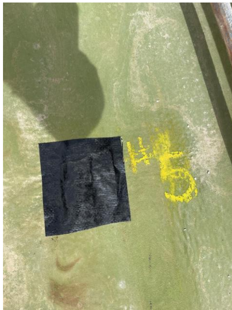
Liner Sample Point #5-patched
