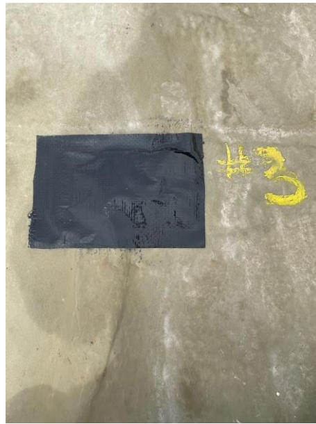
Liner Sample Point #3-patched
