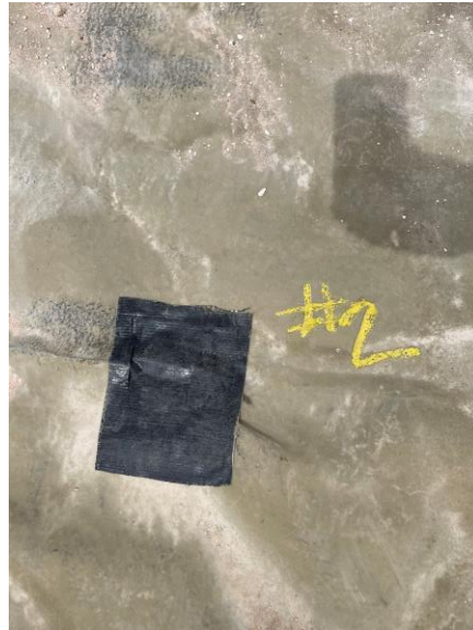
Liner Sample Point #2-patched
