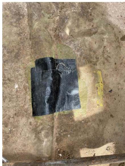
Liner Sample Point #9-patched
