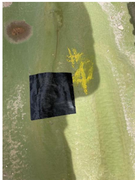
Liner Sample Point #4-patched
