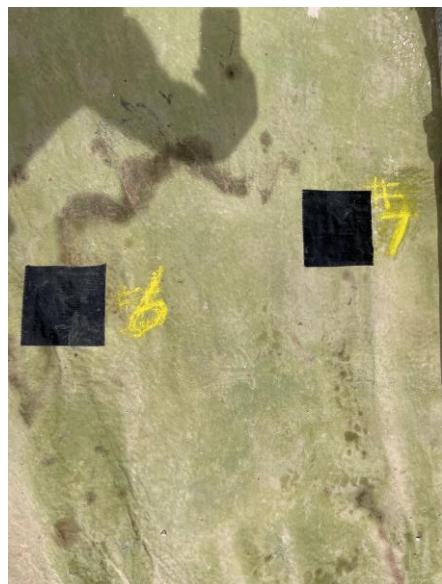
Liner Sample Point #6 and #7-patched
