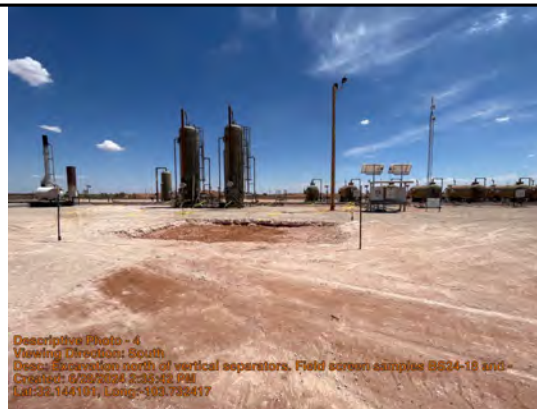
Excavation north of vertical separators. Field screen samples BS24-18 and -21 at 1ft and WS24-06 at 0-1ft
