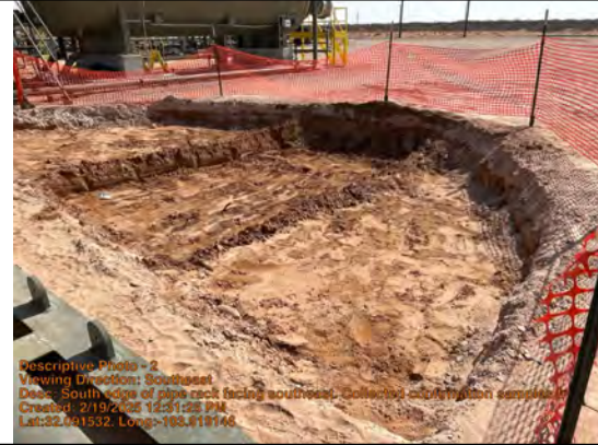
South edge of pipe rack facing southeast. Collected confirmation samples from excavations to 1.5 and 3 feet bgs.
