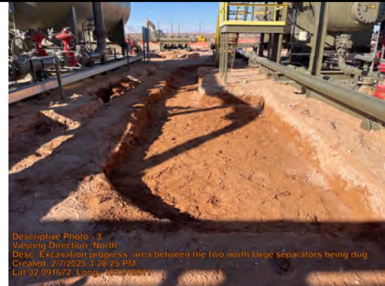
Excavation progress: area between the two north large separators being dug down to 1.5 ft.
