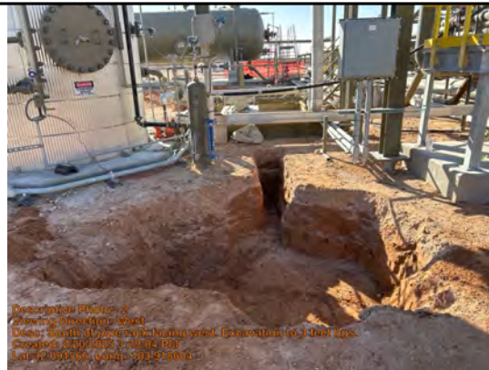
South of pipe rack facing west. Excavation to 3 feet bgs.
