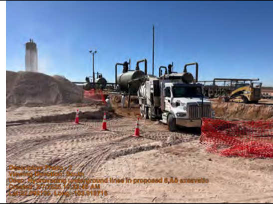
Halo sent out Hydrovac crew to hydrovac around underground lines in proposed 6' excavation.
