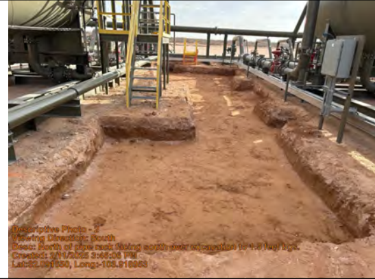
North of pipe rack facing south over excavation to 1.5 feet bgs.
