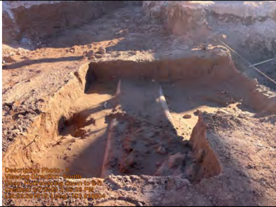
Hydrovacing down to 6 ft
