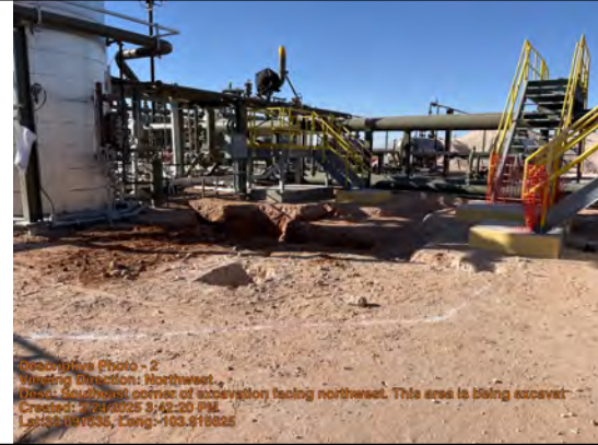
Southeast corner of excavation facing northwest. This area is being excavated using hand tools.
