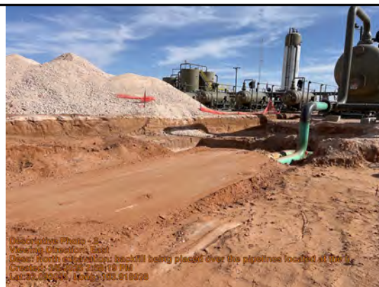
North excavation (24E-04918, nAPP2431846528): backfilling (topsoil) being placed over the pipelines located at the 6ft excavation.
