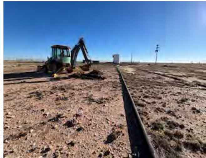
View to S of sample S-18 location.
