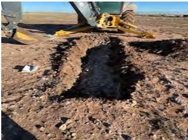
View to SW of sample S-19 location.
