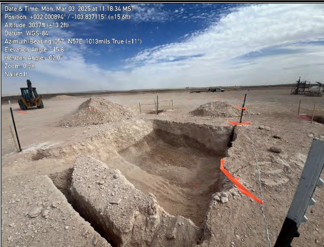
PHOTO 6: Northeastern view of excavation extent. 3/3/2025
