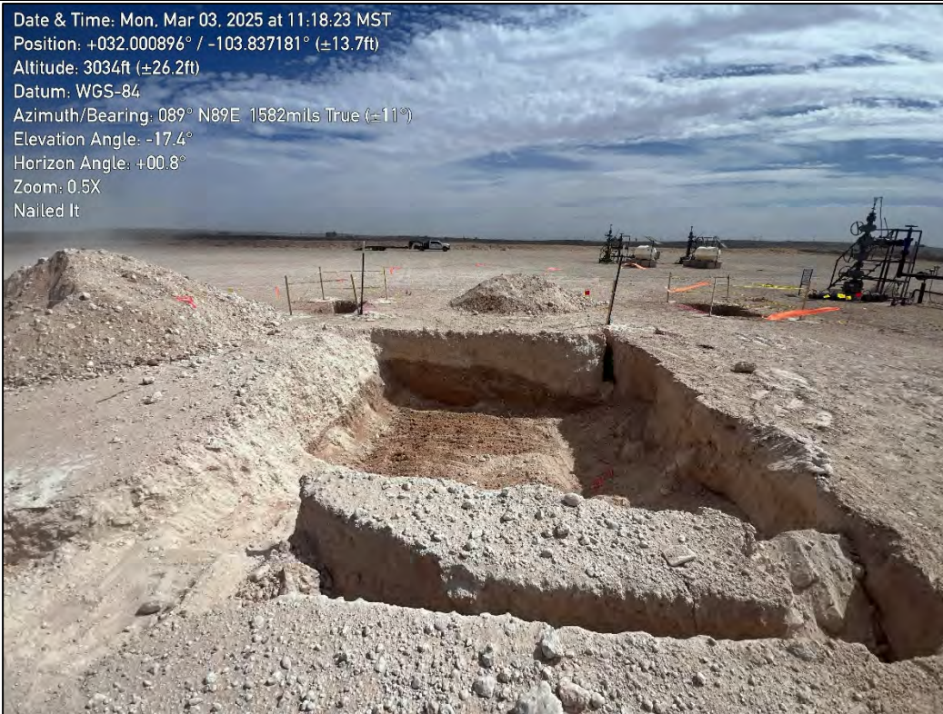
PHOTO 5: Northeastern view of excavation extent. 3/3/2025
