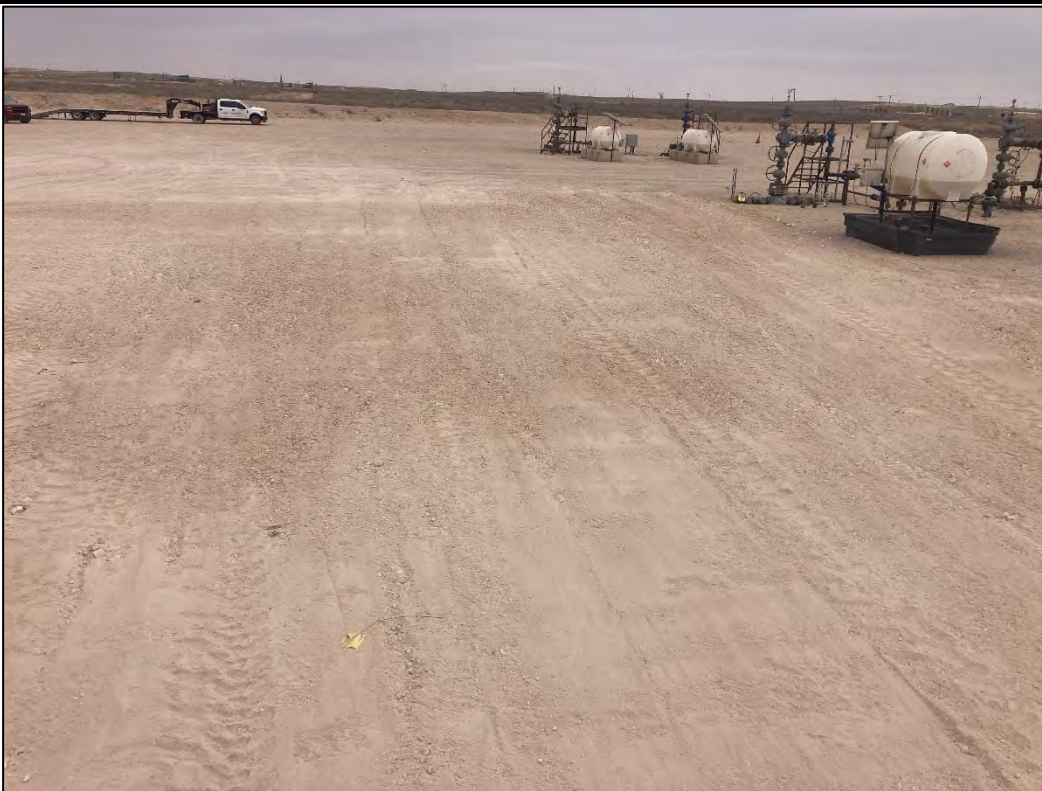
PHOTO 8: Southeastern view following restoration activities. 3/6/2025
