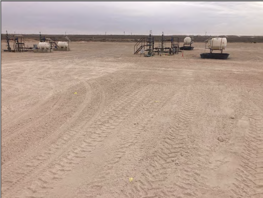
PHOTO 7: Southeastern view following restoration activities. 3/6/2025
