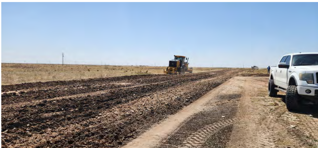
Photograph 40. Equipment ripping up access road leading to the Reed Estate #001 well pad; April 2025.
