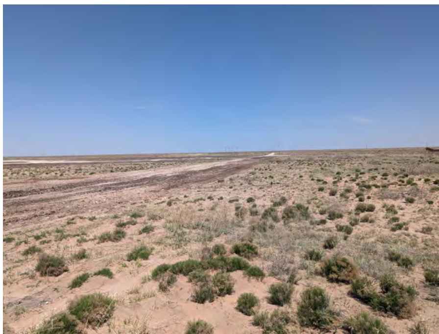
Photograph 41. Reclaimed access road post removal of the top 6-8 inches of caliche then being ripped and seeded; April 2025.
