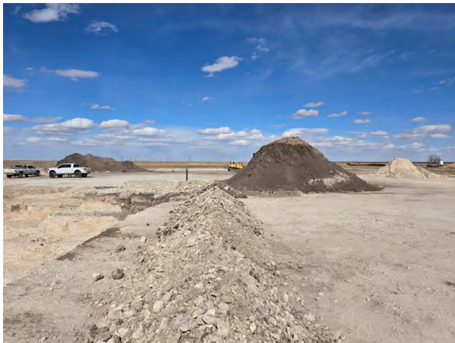
Photograph 21. Looking east at topsoil stockpile adjacent to the Reed Estate #001 well monument along berm placed around southwest excavation for stormwater prevention; January 2025.
