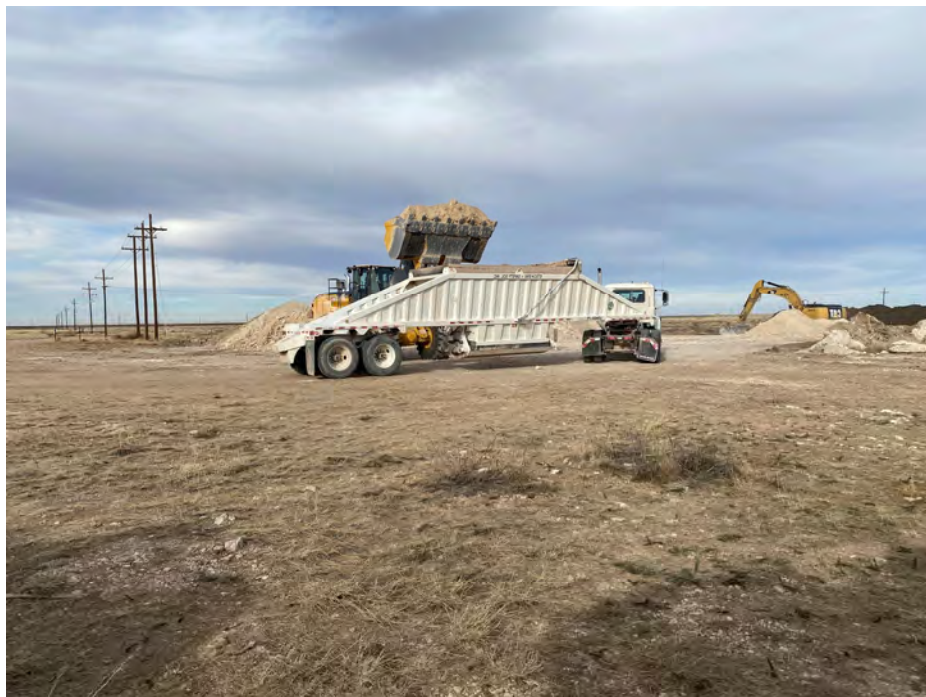
Photograph 3. Front loader filling haul truck with contaminated material to be transported off-site to an OCD-approved disposal facility; December 2023.
