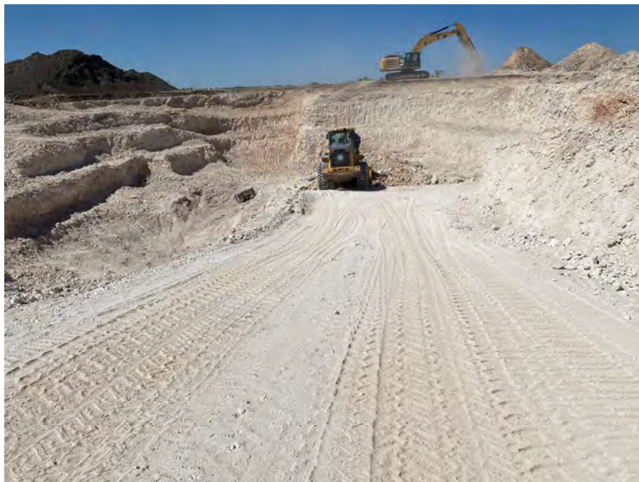
Photograph 11. Looking north along the ramp into the north pit showing front loader removing spoils (foreground), as well as excavator pulling back north benches (background); May 2024.
