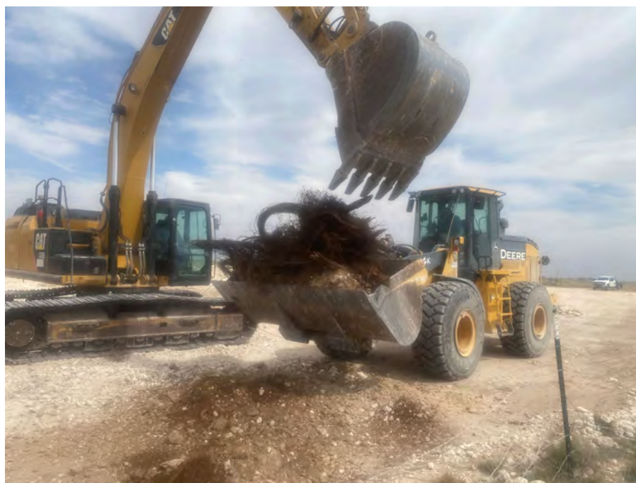
Photograph 10. Front loader transporting debris from a waste pit uncovered during excavation; April 2024.
