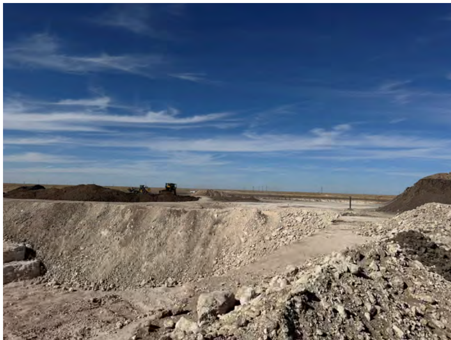
Photograph 31. Backfill progress in the southwest pit near Reed Estate #001 well monument with topsoil stockpile in background to be spread above clean caliche fill across the top 1.5 ft from the surface; March 2025.
