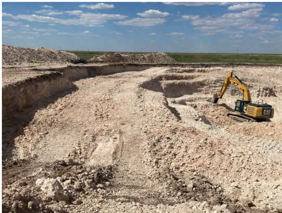
Photograph 13. View looking north at the north pit excavation advancing westward, showing the 5-foot bench along the left (west) edge and overburden stockpiles on the ground surface; September 2024.
