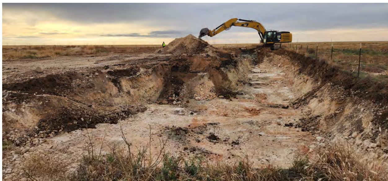
Photograph 2. Excavation along the northern fence/edge, reaching a depth of 4 feet. Dark topsoil is visible at the top 1-1.5 feet, as well as dark hydrocarbon staining below the former tank battery; November 2023.
