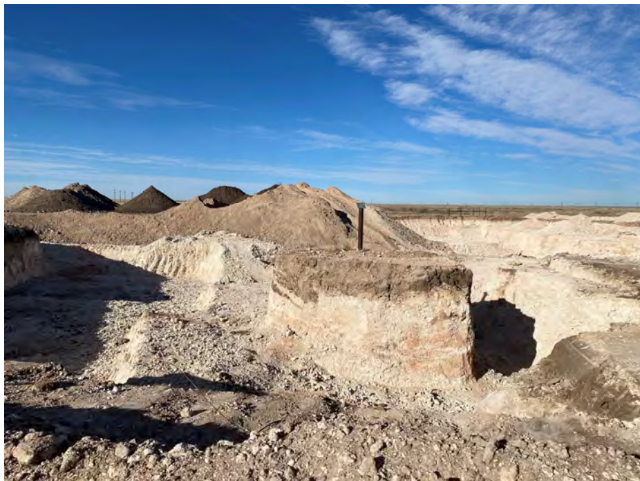
Photograph 5. View looking north toward the Reed Estate #001 well monument, showing a 10-foot radial buffer in place prior to commencement of backfill activities. February 2024.
