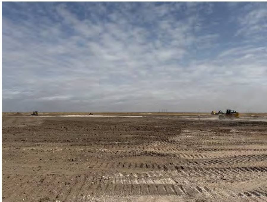
Photograph 36. UC2 shaping final grade across recently placed topsoil in the northeast section of the site; April 2025.
