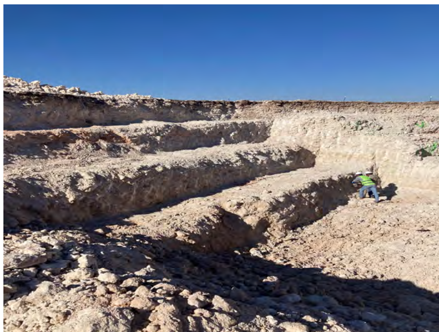
Photograph 16. View of the northwest benches of the north pit at geologists collecting soil samples of the bottom 5-ft bench with hammer drill (standing approximately 20 feet below ground surface); October 2024.
