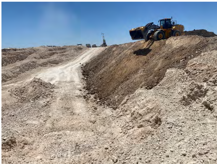
Photograph 12. View looking south at the front loader placing backfill on the northeast side of the north pit after passing closure criteria; May 2024.
