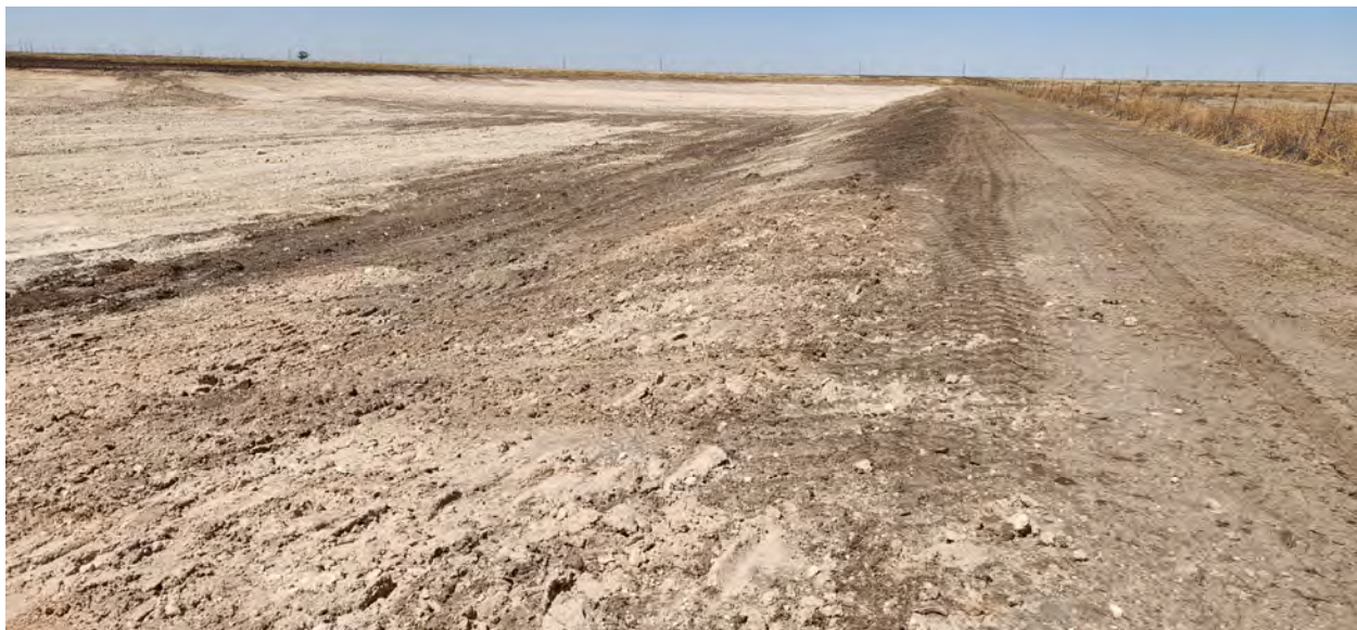
Photograph 33. Looking west along northern edge of borrow area showing compliance with requests from landowner for 3:1 slopes and a minimum 15-ft off-set from north fence line.
