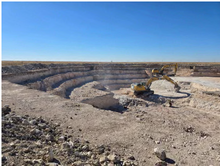
Photograph 19. Looking west into the southwest pit at excavator removing material from the pit floor. Berms placed around the excavation to keep stormwater out of excavation; January 2025.
