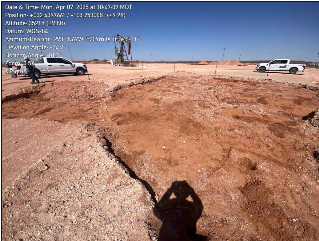
PHOTO 21: Northwestern view of excavation extent. 4/7/2025
