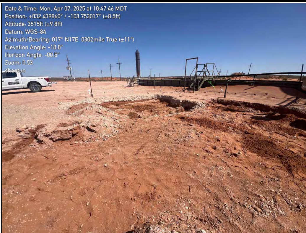
PHOTO 20: Northeastern view of excavation extent. 4/7/2025
