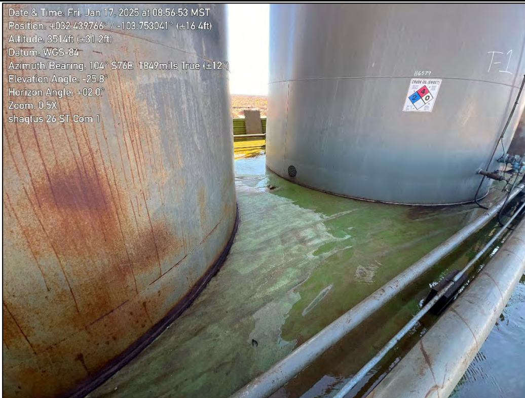
PHOTO 13: Southeastern view during liner inspection activities. 1/17/2025
