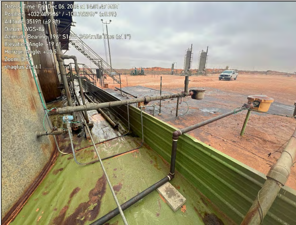
PHOTO 1: Southwestern view during initial site assessment activities. 12/6/2024
