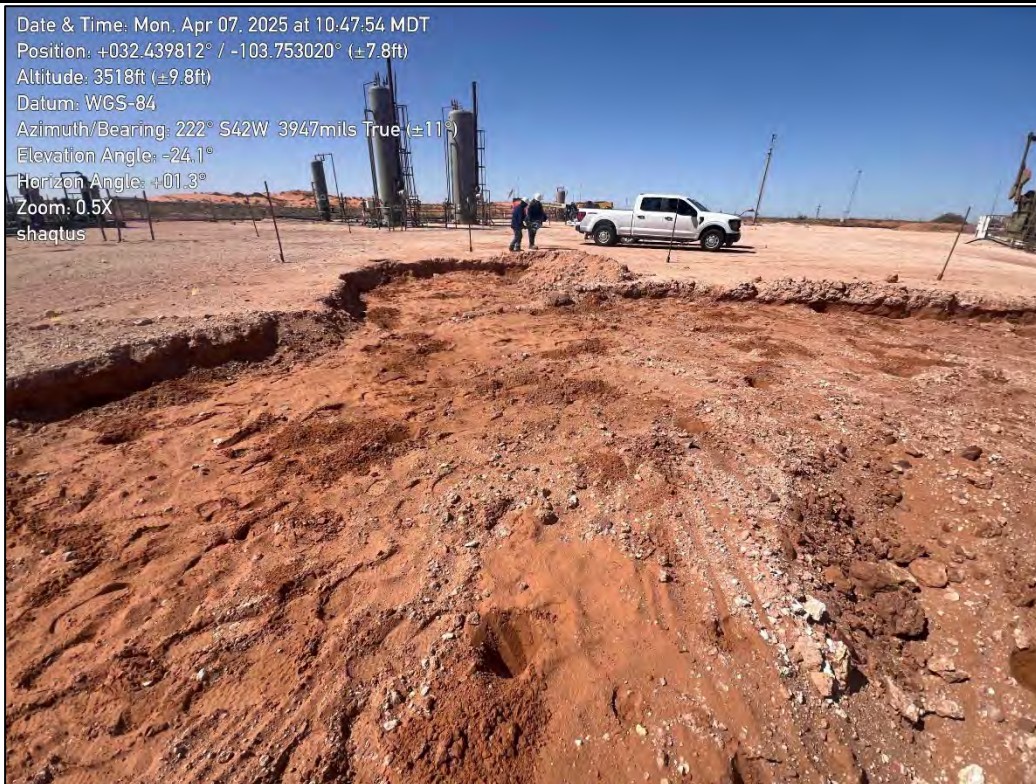
PHOTO 19: Southwestern view of excavation extent. 4/7/2025
