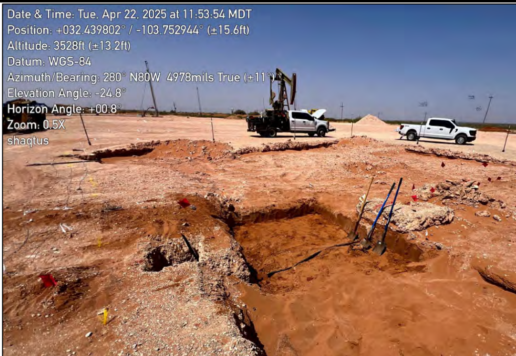
PHOTO 22: Northwestern view of excavation extent. 4/22/2025
