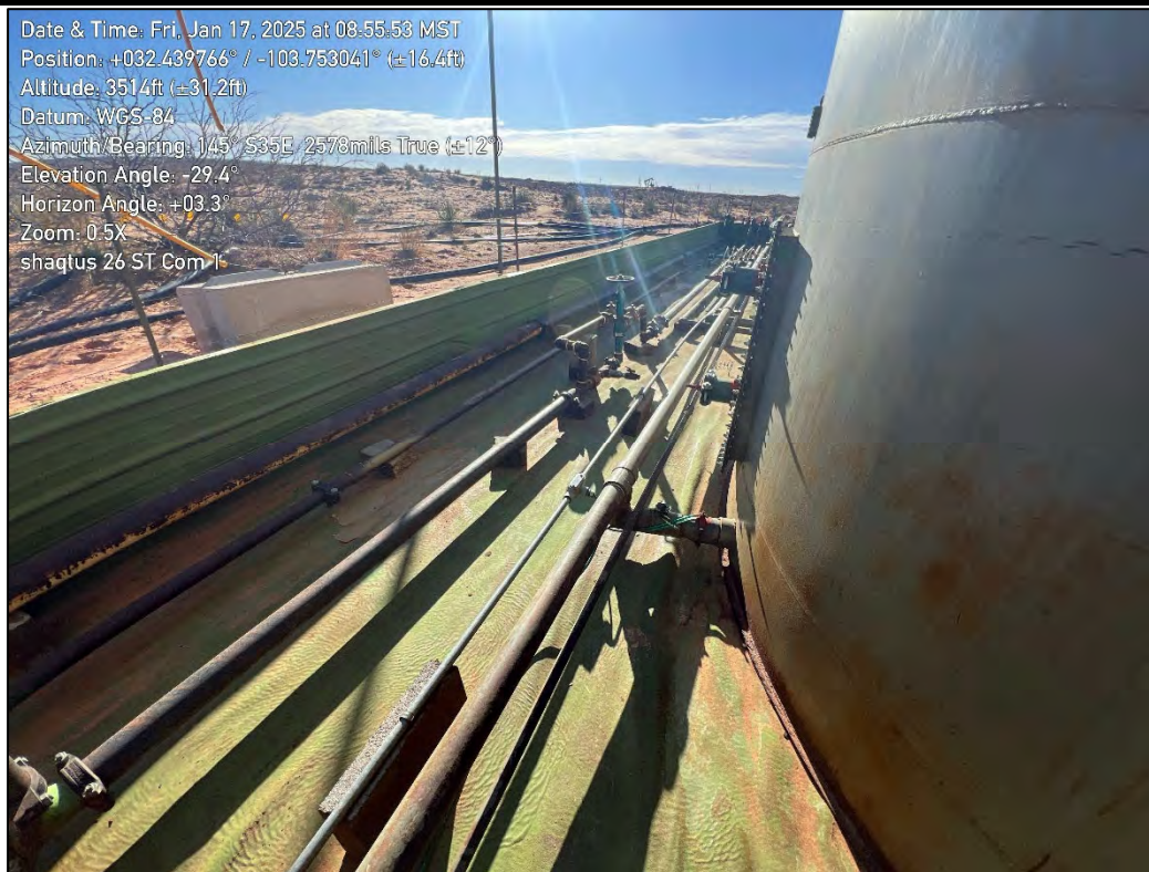
PHOTO 11: Southeastern view during liner inspection activities. 1/17/2025
