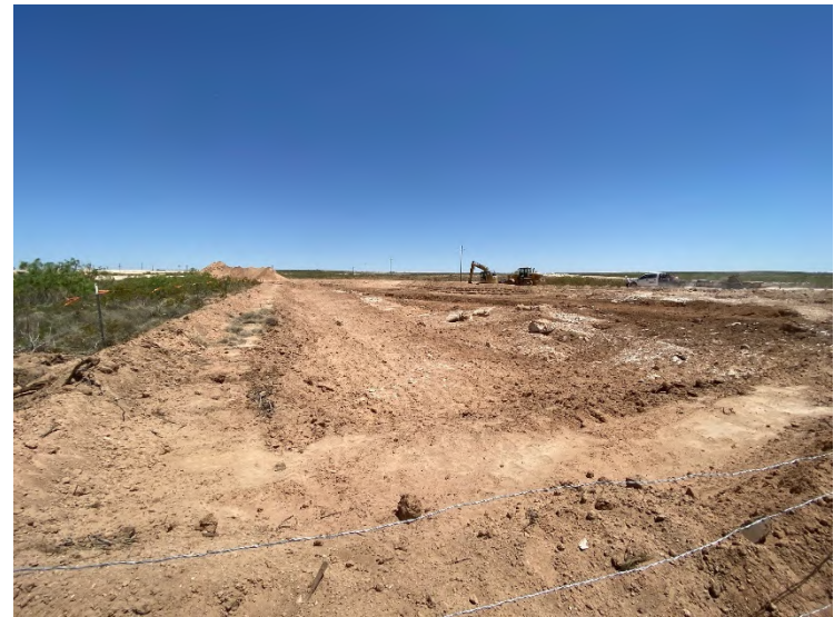
Photograph 4: Eastern view during excavation activities.
