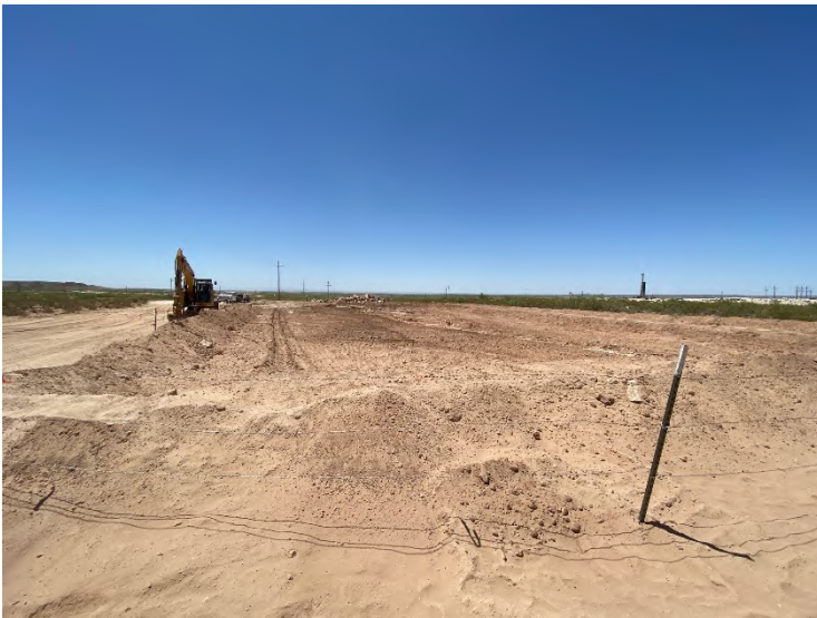
Photograph 3: Western view during excavation activities.
