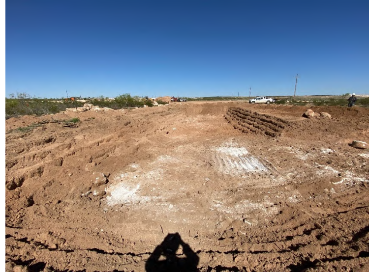
Photograph 2: Eastern view during excavation activities.
