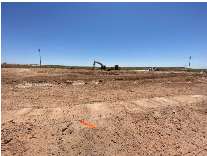
Photograph 5: Southern view during excavation activities.
