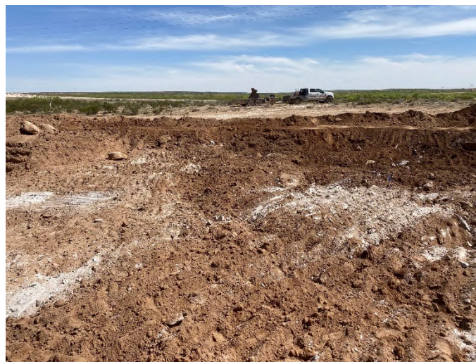
Photograph 6: Southern view during excavation activities.
