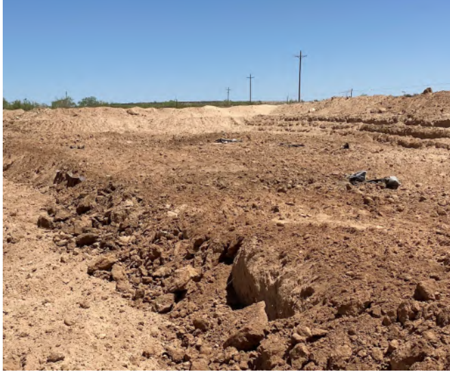
Photograph 1: View of exposed liner.
