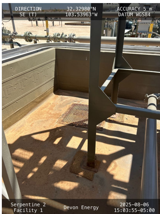
Photo 13 View of southeast corner of secondary containment.
