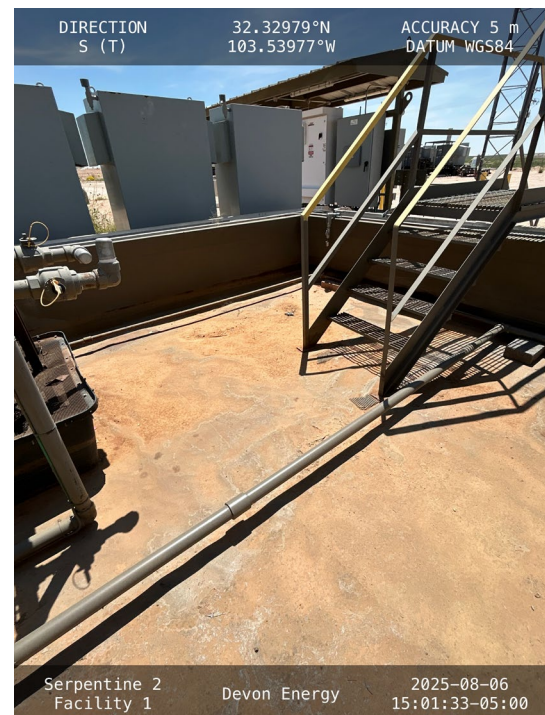
Photo 2 View of southeast corner of secondary containment.
