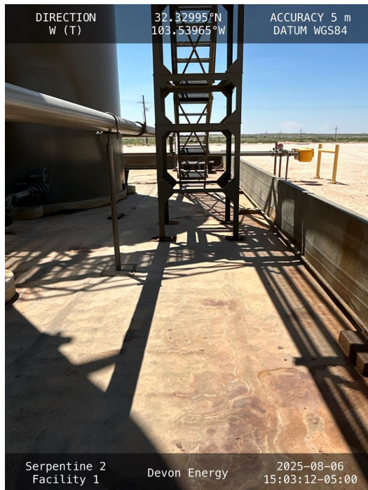
Photo 9 View of northern portion of secondary containment facing west.
