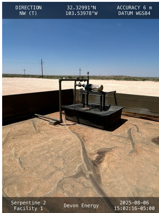
Photo 5 View of northwest corner of secondary containment.
