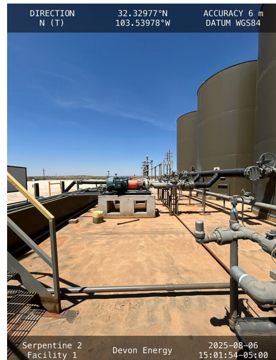
Photo 4 View of western portion of secondary containment facing north.
