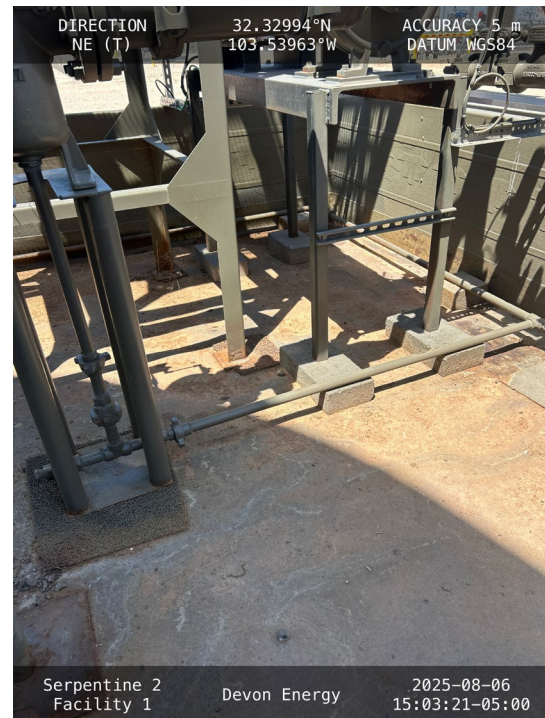
Photo 10 View of northeast corner of secondary containment.
