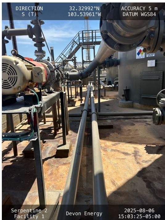
Photo 11 View of eastern portion of secondary containment facing south.
