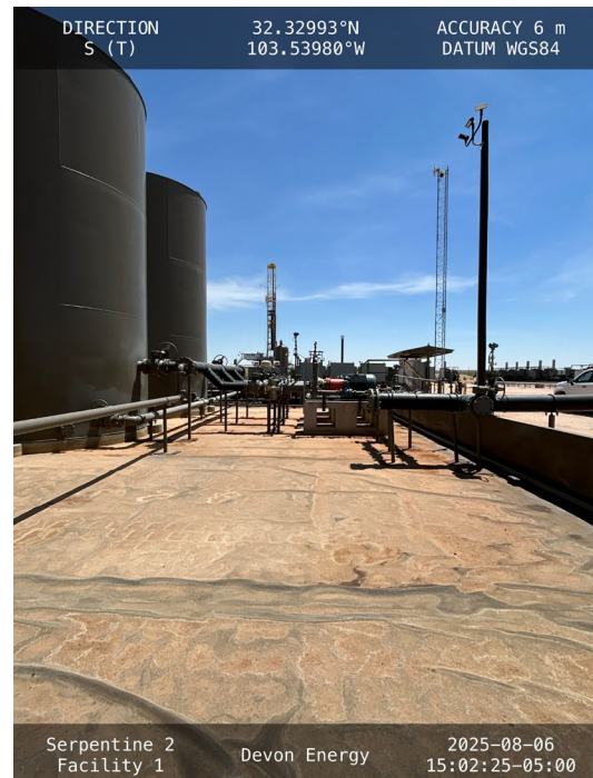
Photo 6 View of western portion of secondary containment facing south.
