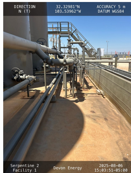
Photo 12 View of eastern portion of secondary containment facing north.
