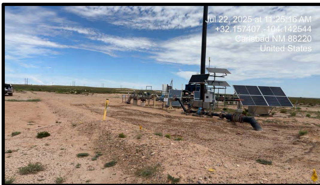
PHOTOGRAPH NO. 1 – A view of the impact/remediation area upon completion. The view is towards the north.
