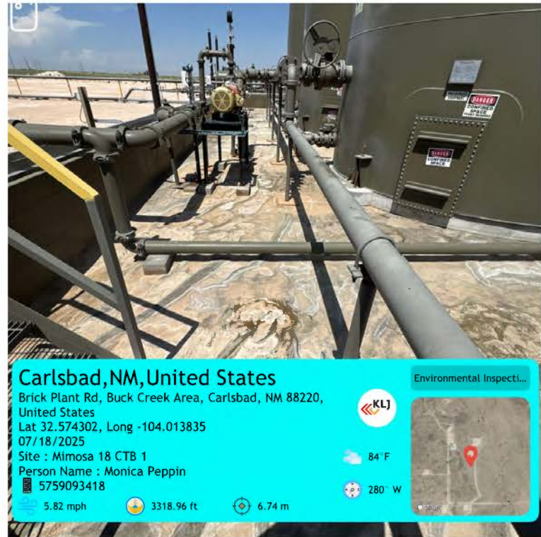
South end of containment facing west
