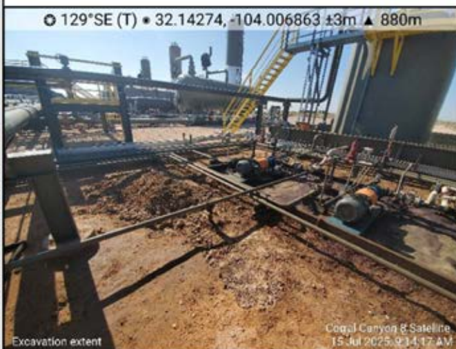
Photograph: 10 Date: 07/15/2025 Description: Hand excavation activities near the lined containment View: Southeast
