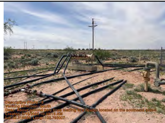
Above ground poly lines leading to a header located on the southeast side of the deferral area.
